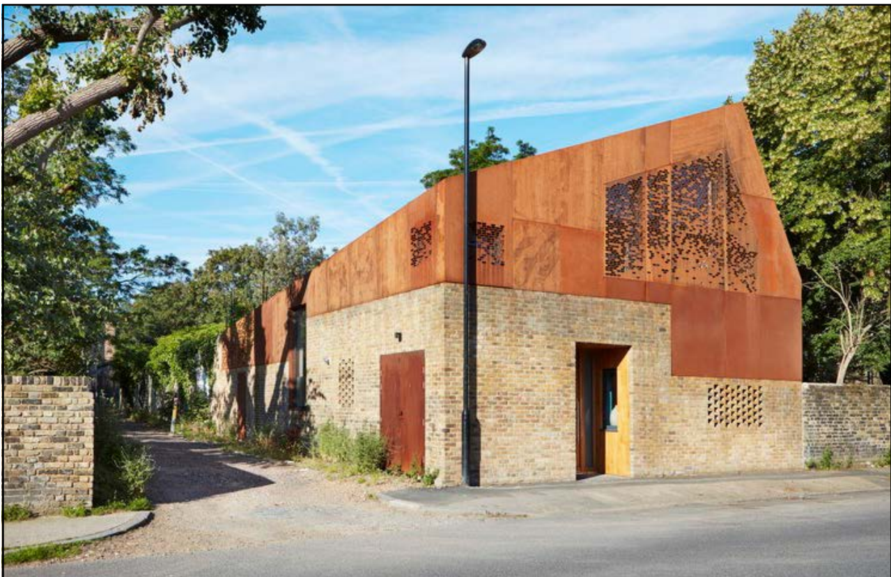
Fig. 129: This new house by Stolon Studio cleverly utilises a site at the entrance to an existing mews to create an attractive family home. The front door is set back from the pavement and ground floor windows use hit-and-miss brickwork to provide privacy. (website: www.stolon.co.uk , photography: Paul Murphy)
