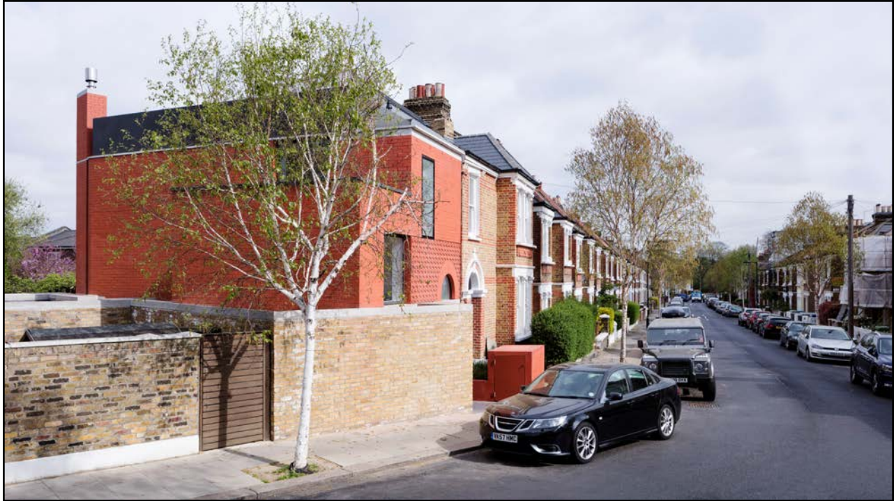
Fig. 127: Respecting the height and detail of the neighbouring houses, this new family home by 31/44 architects extends an existing Victorian terrace in Southwark. (website: www.3144architects.com , photography: Rory Gardiner)
