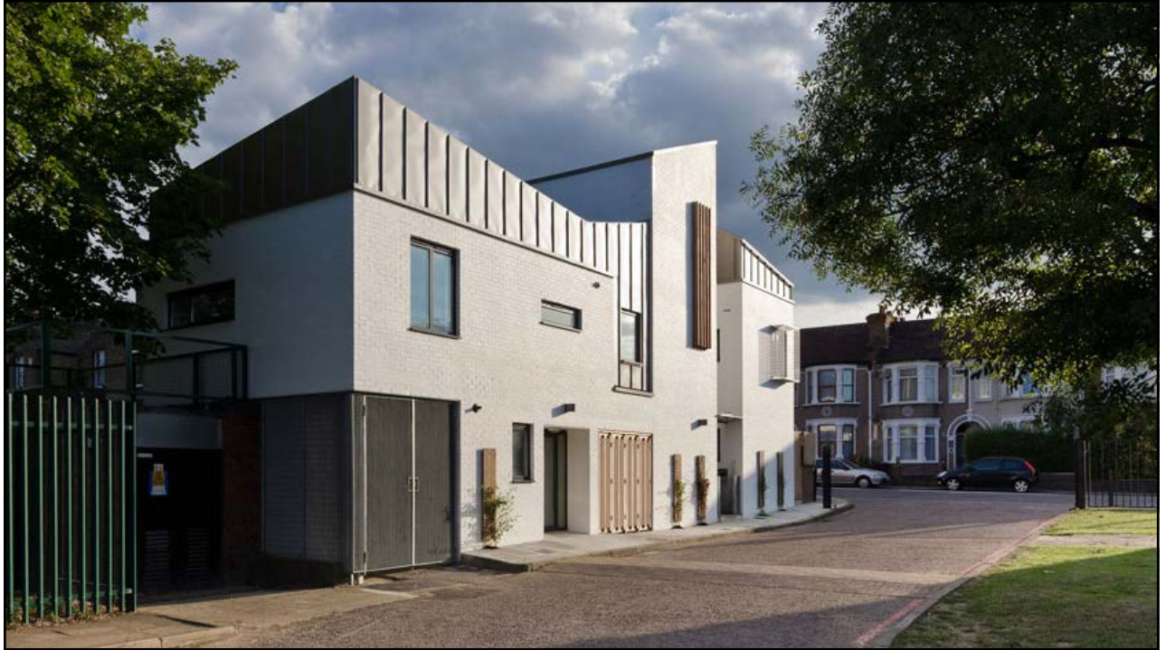
Fig. 142: The small residential development on the corner of two streets in Crofton Park replaces a school keeper's cottage with three flats and a small house. (website: www.chancedesilva.com , photography: Tim Crocker)
