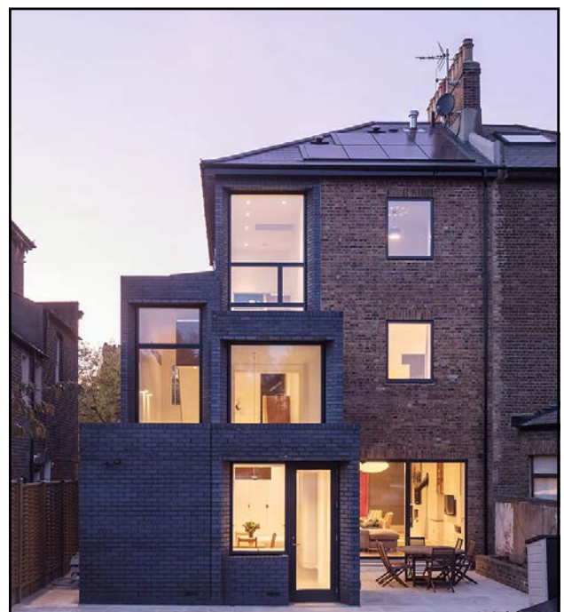
Fig. 82: This new house in Brockley Conservation Area, designed by Gruff Architects, was a complete re-build of the former non-historic building on the site. This new house carefully replicated the detail of the adjacent historic group, reinstating the original uniformity. At the rear, the development is successful in responding to the building line, pattern of extensions, and fenestration arrangement of the adjacent historic buildings in a contemporary language (website: gruffarchitects.com , photography: Simon Kennedy)
