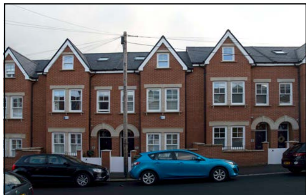
Fig. 111: New homes in Crofton Park designed by Brooks Murray Architects. (website: www.brooksmurray.com , photography: RCKa)
