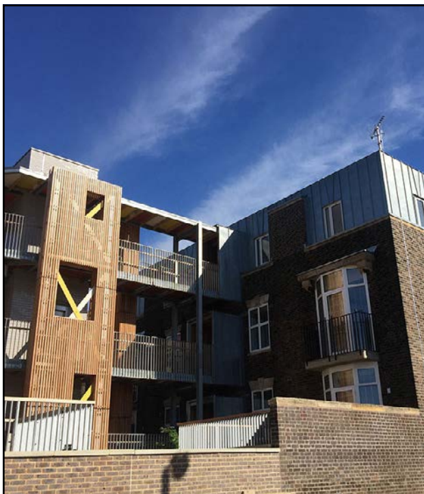
Fig. 163: The refurbishment and vertical extension of St Paul's House in Deptford by Ash Sakula (website: www.ashsak.com , photography: Ash Sakula)
