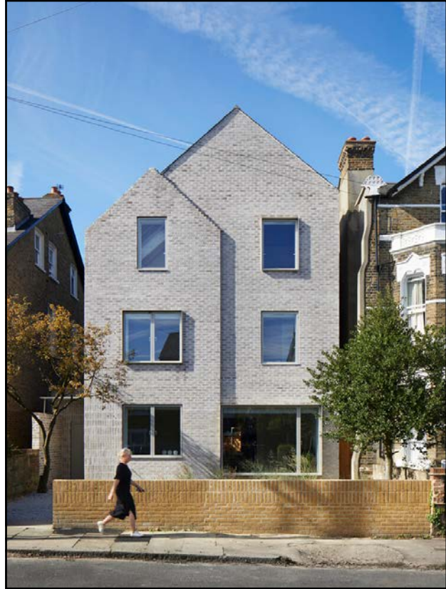
Fig. 185: Vertical extension and recladding of an existing house following the principles of street infill development. Designed by alma-nac (website: www.alma-nac.com , photography: Jack Hobhouse).
