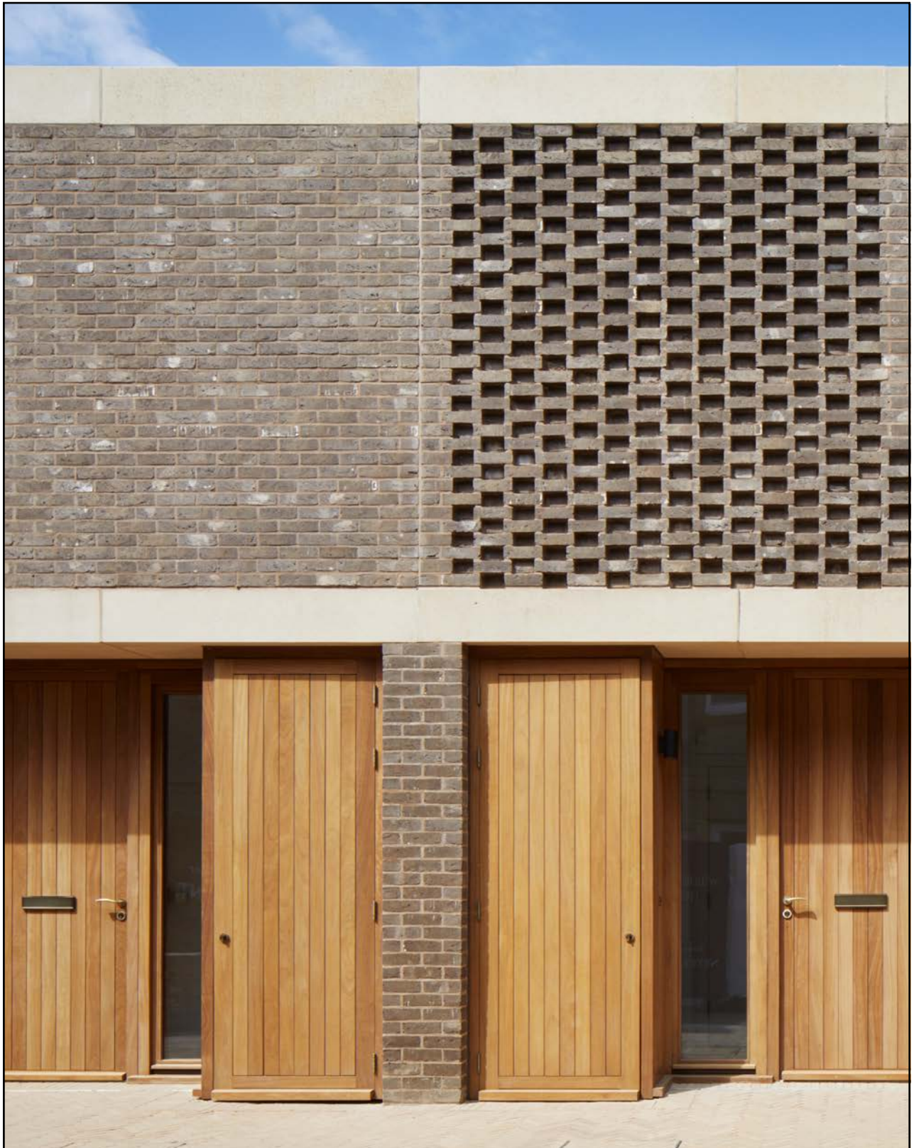
Fig. 34: These new mews houses in Sevenoaks, designed by Morris + Company, smartly integrate waste storage into the building envelope, providing a more friendly and usable public realm (website: www.morrisandcompany.com , photography: Jack Hobhouse)
