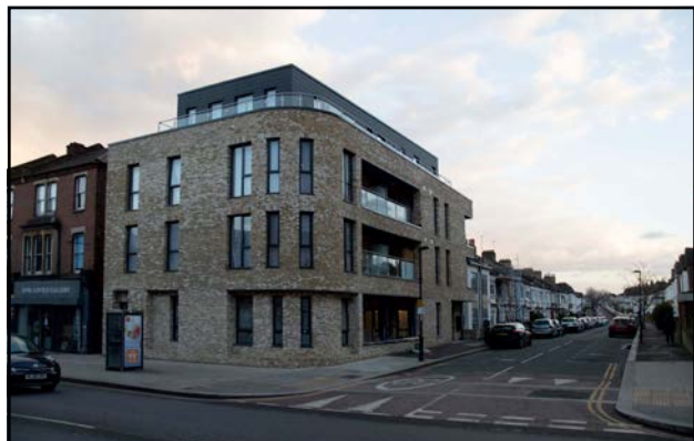
Fig. 141: Corner development in Sydenham
