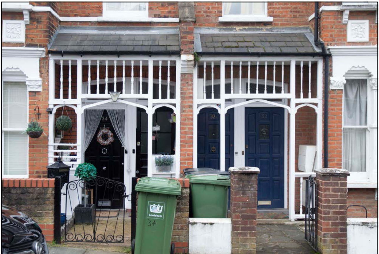
Fig. 35: ‘Walk up’ houses on Chalsey Road. Four houses, each with their own front doors, but two houses have most of their accommodation on the upper floors. (photography: RCKa)
