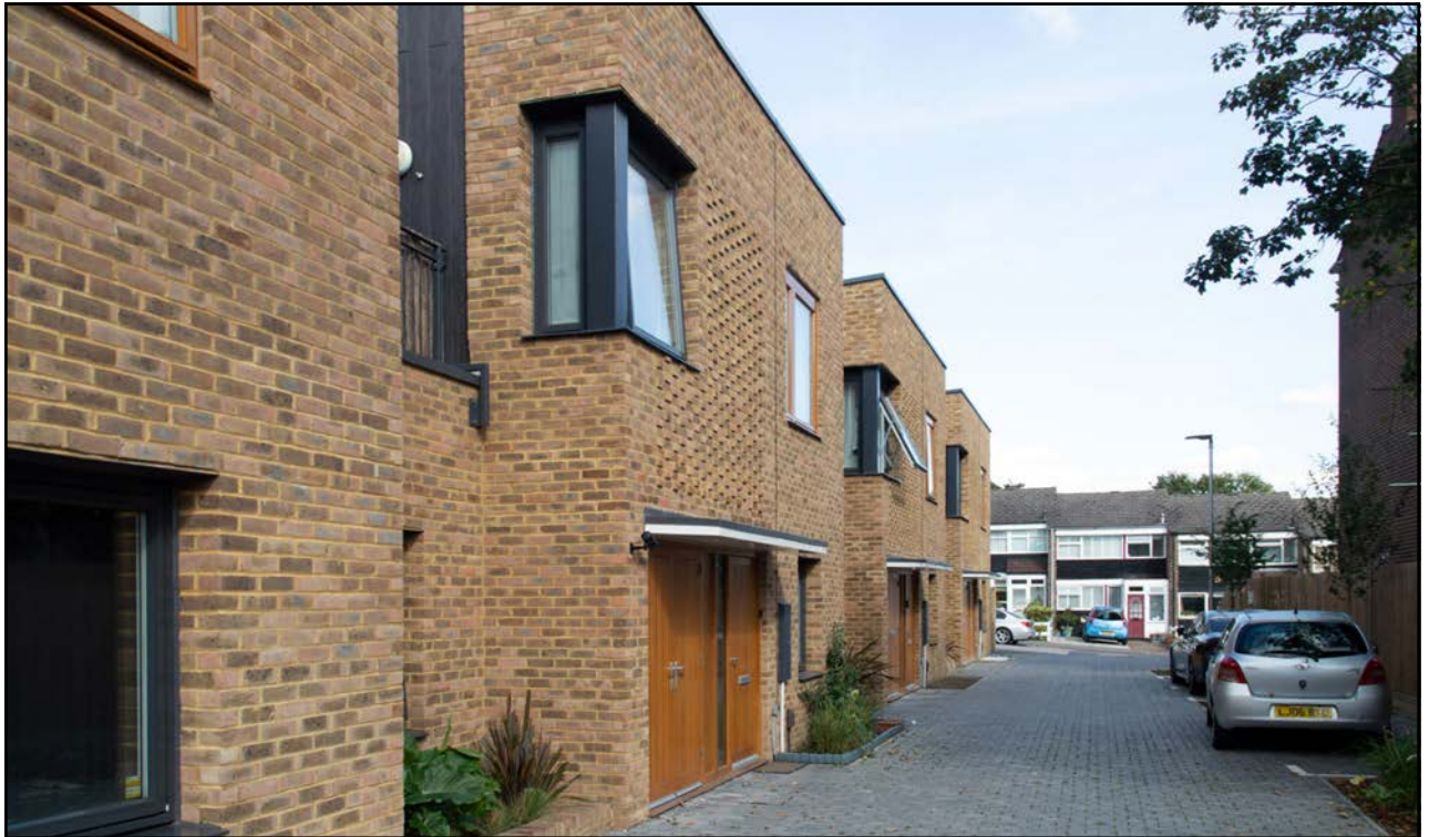
Fig. 14: New homes at Dacre Park in Lee designed by Pollard Thomas Edwards Architects (website: www.pollardthomasedwards.co.uk , photography: RCKa)
