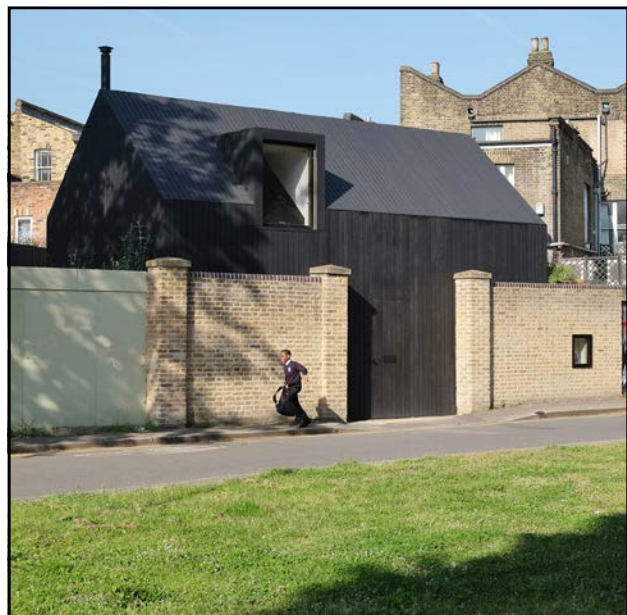
Fig. 151: New house facing St Paul's church in Deptford designed by Jonathan Pile. (website: www.oval-uk.com , photography: Gareth Gardner)
