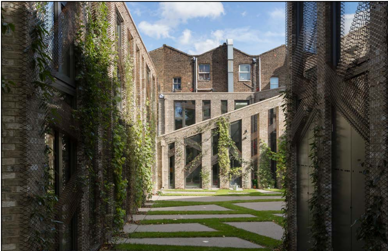
Fig. 36: Access into Forest Mews, designed by Stolon Studio, is via a private road which allows soft landscaping to be integrated into the vehicular access (website: www.stolon.co.uk , photography: Robert Barker)
