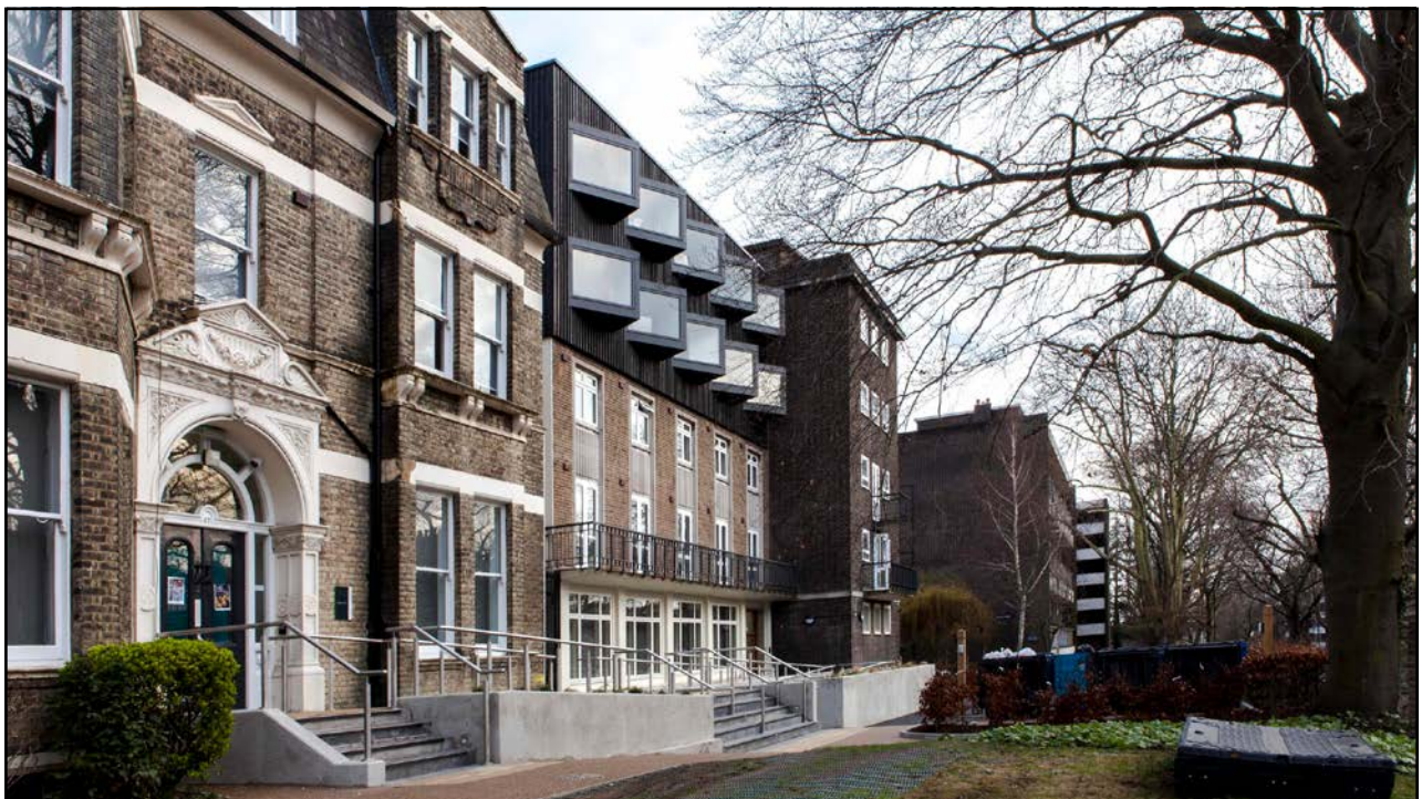
Fig. 161: Extension to Raymont Hall by Hawkins\Brown providing new student accommodation. (website: www.hawkinsbrown.com , photography: Francesco Montaguti)
