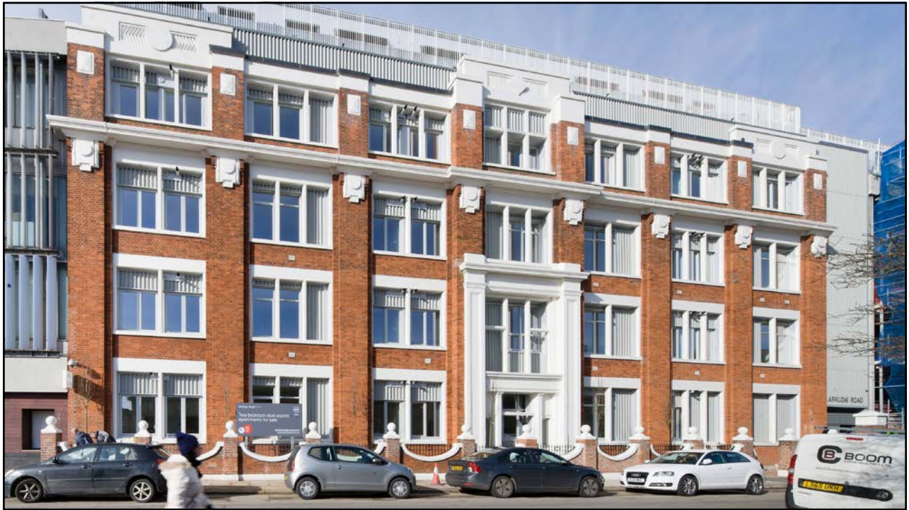
Fig. 160: The refurbishment and vertical extension of Astra House in New Cross by RCKa provides new dual-aspect residential accommodation through the intensification of a formal commercial building. (website: www.rcka.co.uk , photography: Jakob Spriestersbach)
