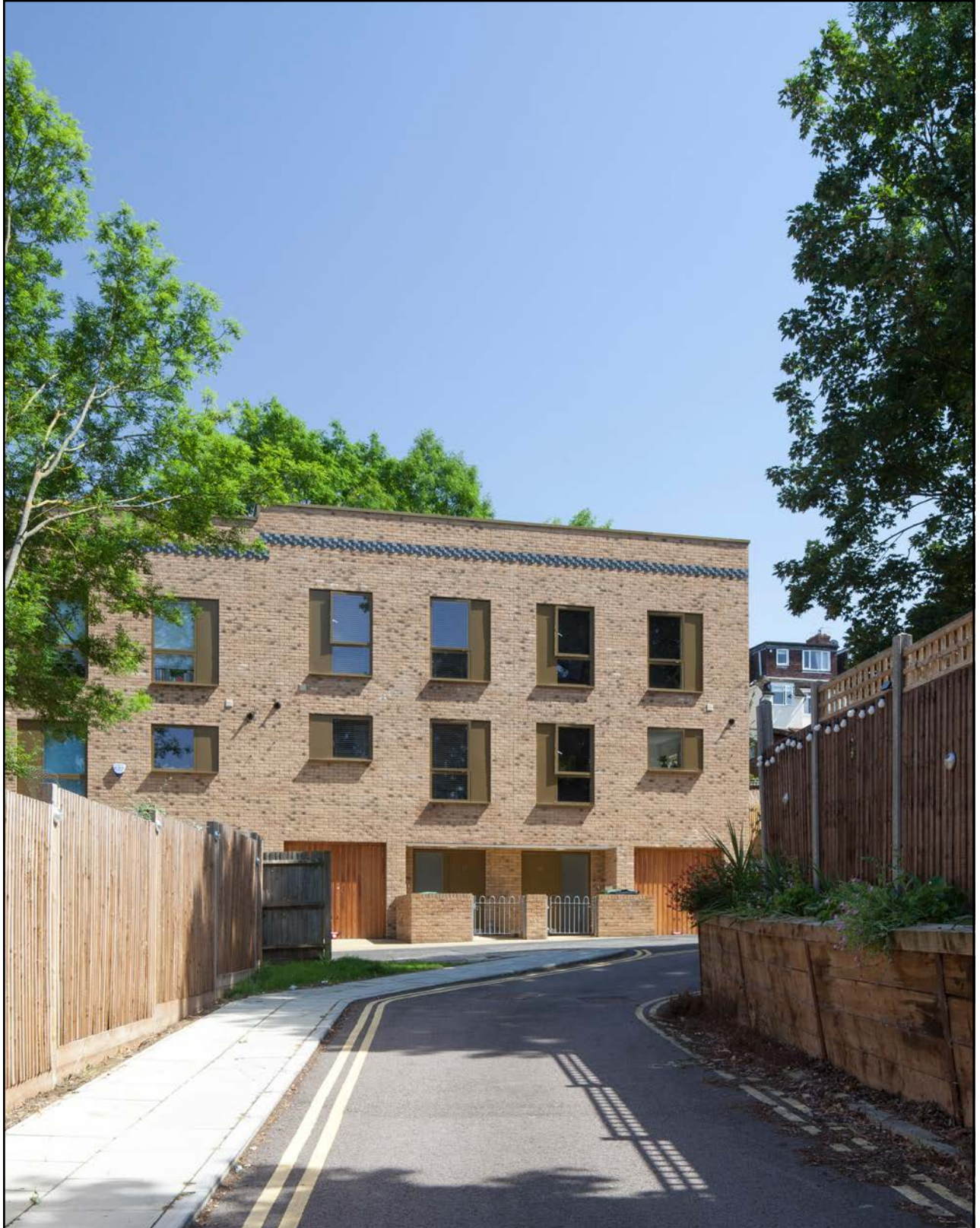
Fig. 96: New homes in Forest Hill designed by David Miller Architects (website: www.david-miller.co.uk , photography: Agnese Sanvito)
