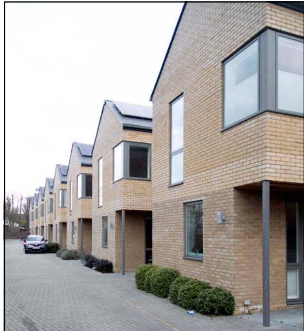
Fig. 168: 8 new homes in Crofton Park designed by Inhouse Design Associates Architects (website: www.inhousearchitects.co.uk , photography: RCKa)
