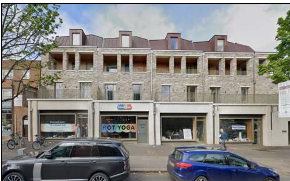
Fig. 164: Vertical intensification in Southwark designed by Panter Hudspith (website: www.panterhudspith.com , photography: Panter Hudspith)
