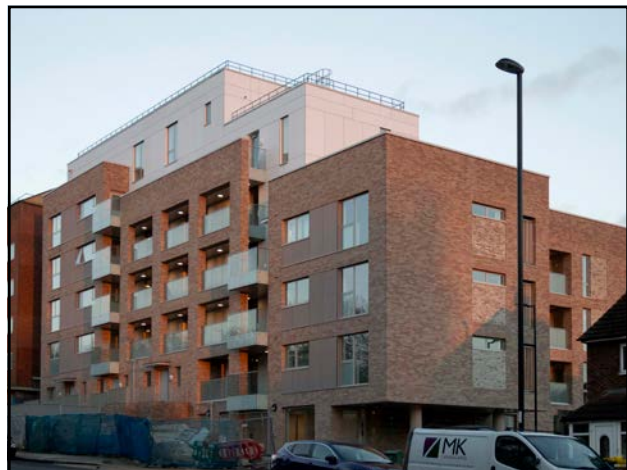
Fig. 107: Forster House in Whitefoot designed by Levitt Bernstein Architects (Website: www.levittbernstein.co.uk , Photography: RCKa)
