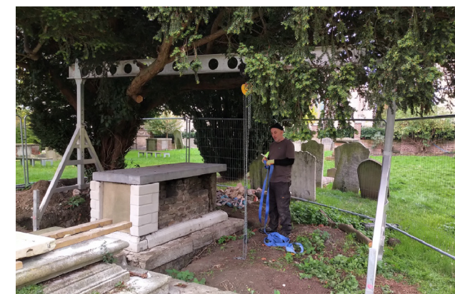
Photo 5: Dismantling the grade II Butler tomb, St Margaret's Old Churchyard
