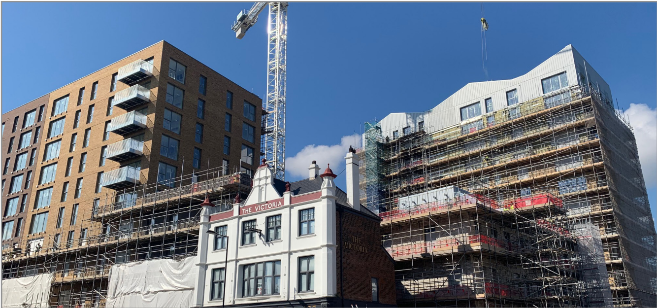
Photo 6: Timberyard under construction Source: LB Lewisham
