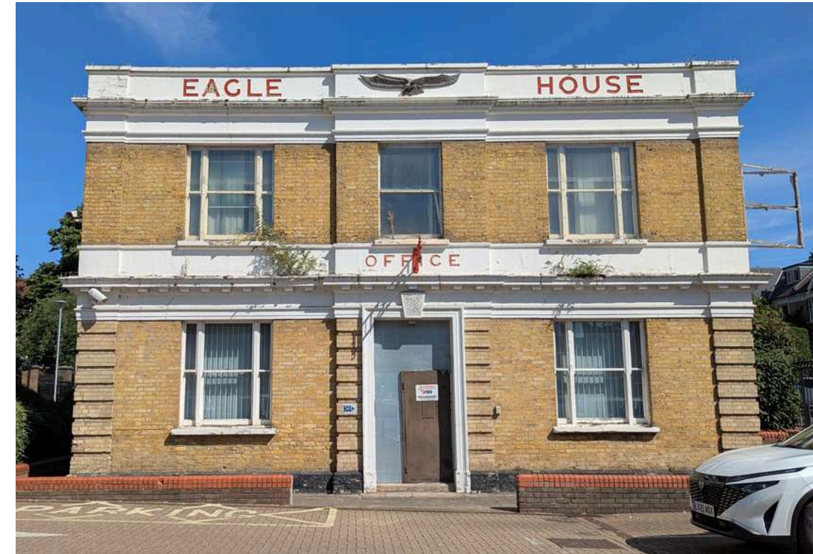
Eagle House, the only remaining building of the Anchor Brewery
