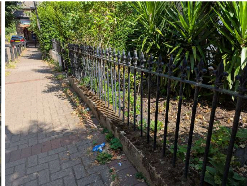
Possible original railings on Silk Mills Path
