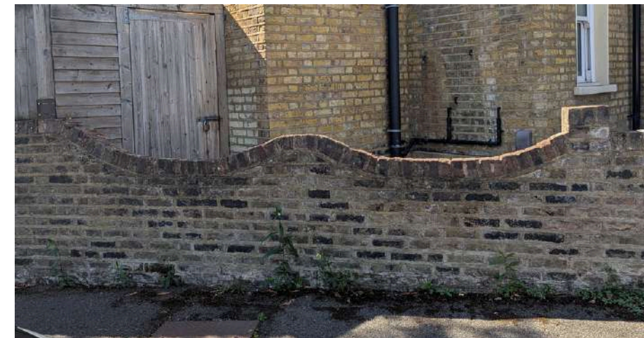
Possibly original boundary wall in Sunninghill Rd.
