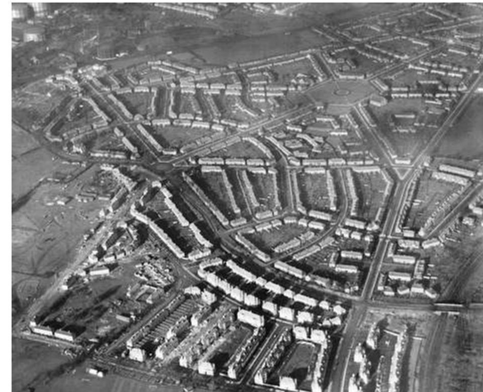
Aerial photograph of Bellingham Estate, 1937. The second phase south of Southend Lane is mostly constructed. Source: Britain from Above, EPW056116
