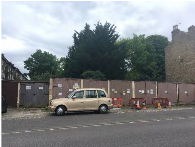
Garages, Wisteria Road, SA05
