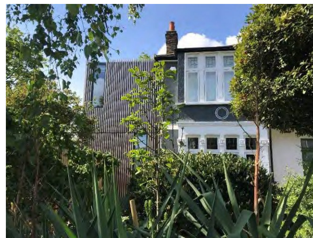
Right. Manor Park, Lee Forum area. Use of starkly contrasting geometry, materials and fenestration does not attempt to create an extension, rather an addition of the original house, from which the addition is clearly legible. Although the materials are not typical of the area, the use of timber softens the impact and fits in well with the mature landscaping and the riverside location. R2 Studio Architects
