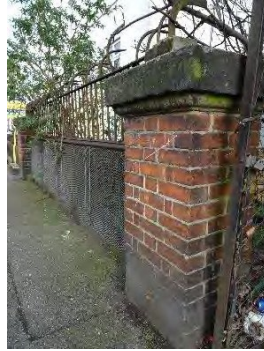
Bridge, Eastdown Park
