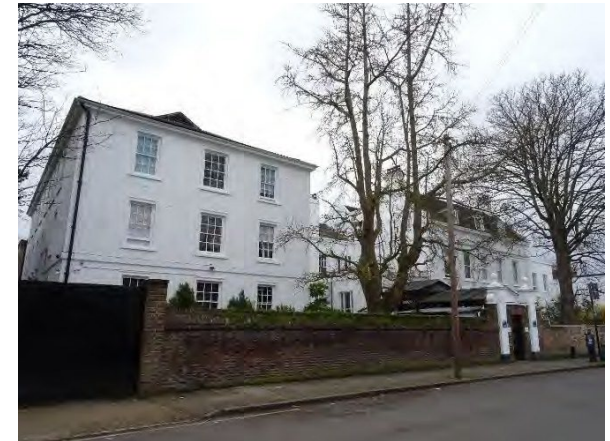
Grade II listed Pentland House and Glencorse House, Old Road
