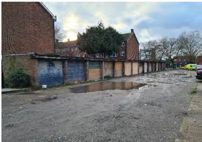
Garages off Burnt Ash Road, SA09
