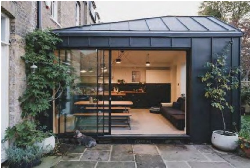
Above. Micheldever Road, Lee Forum area. This addition is read clearly alongside and without detriment to the original property. The forms respect the neighbouring properties and rear first floor windows. The geometry is accentuated by the folded sheet zinc, creating clean lines, contrasting with the original building. Meme Architects
