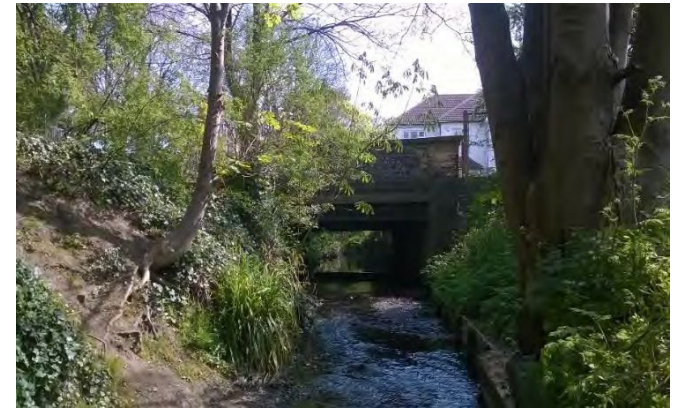
River Quaggy, Weigall Road bridge
