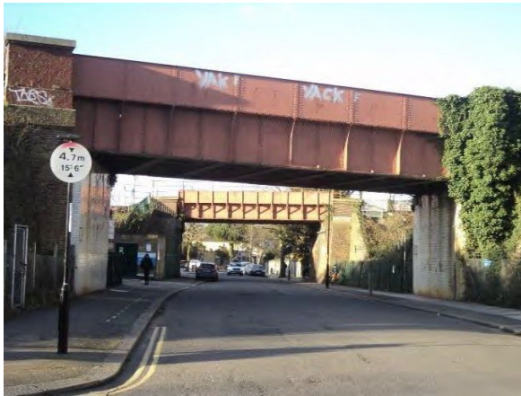
Two railway bridges at Manor Lane
