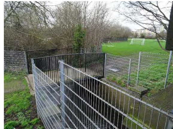
Bridge over the River Quaggy, John Roan Sports Club
