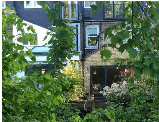
Rear extension from Manor Park
