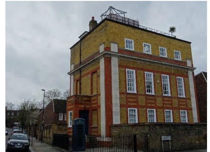
Above. cnr Gilmore Rd and Eastdown Park, Lee Forum area. Old Telephone Exchange. Grade II Listed building converted to residential whilst preserving the original external envelope. Blends contemporary elements such as glazed metal framed screens with original features. Flat roof has been transformed to a sun terrace. The Gilbert Scott designed telephone box previously stood outside the property, now stands next to the entrance housing a light sculpture.
