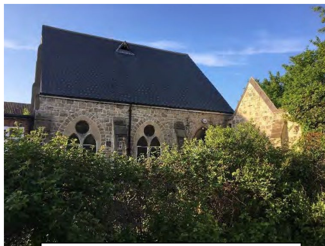
United Reformed Church, Burnt Ash Road
