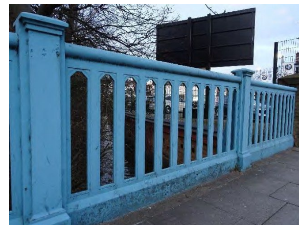
Bridge over River Quaggy, Lee High Road
