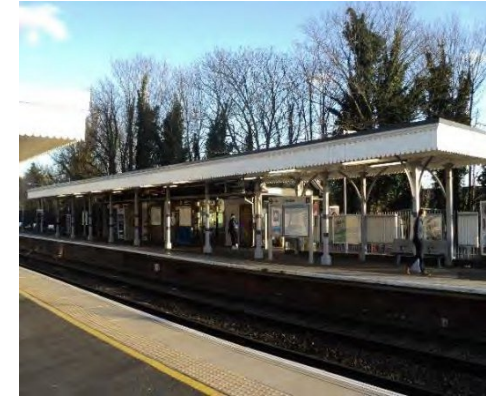
Platform 1, Lee Railway Station
