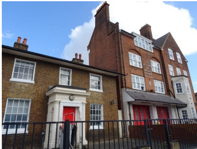
Fire Station, Eltham Road
