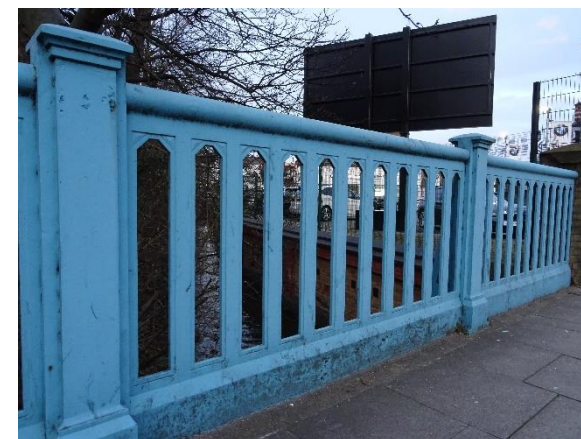
Bridge over River Quaggy, Lee High Road
