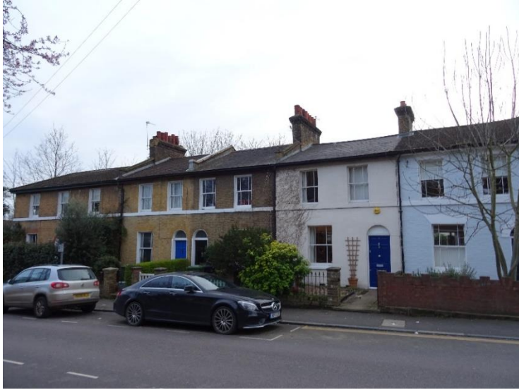
Surviving row of cottages in Dacre Park
