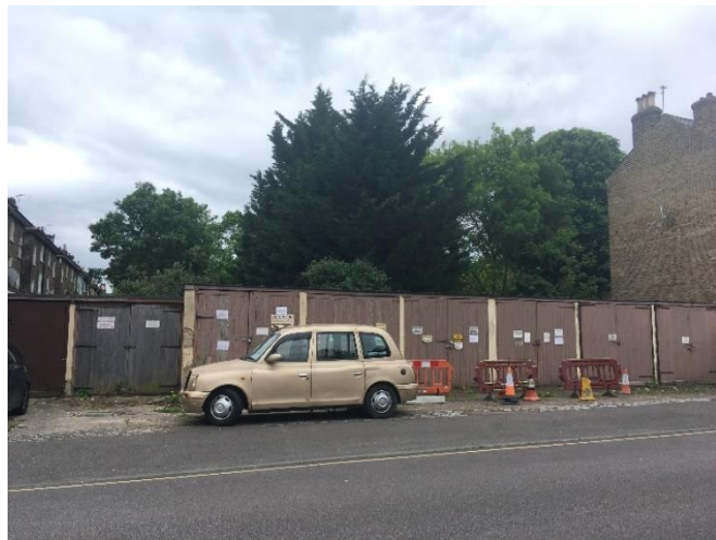
Garages, Wisteria Road, SA05
