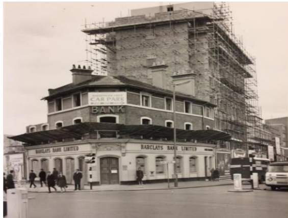
Lee Green Crossroads, towards Burnt Ash Road
