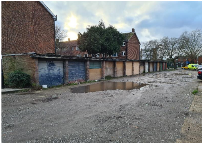
Garages off Burnt Ash Road, SA09
