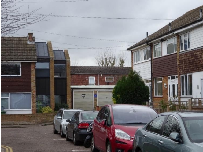
Left. Wolfram Close, Lee Forum area. The staggered forms of this two storey extension and change of materials distinguish it from the original building. Details like the cast concrete pads and gutter zinc gives a streamlined finish. The 2 sections of the recessed extension, set back from the public realm, do not intrude on the eye or the surrounding space and nearby dwellings, but blend in. The development allows for small front garden spaces and synchronicity with the original house. Selencky /// Parsons Architects
