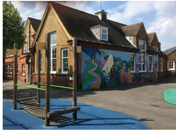
2. Community Infrastructure (Brindishe Lee School, Leahurst Road)
