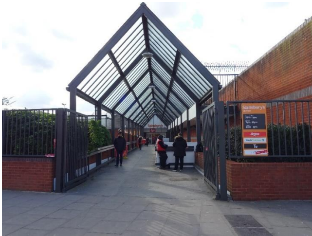
Sainsbury's, Burnt Ash Road
