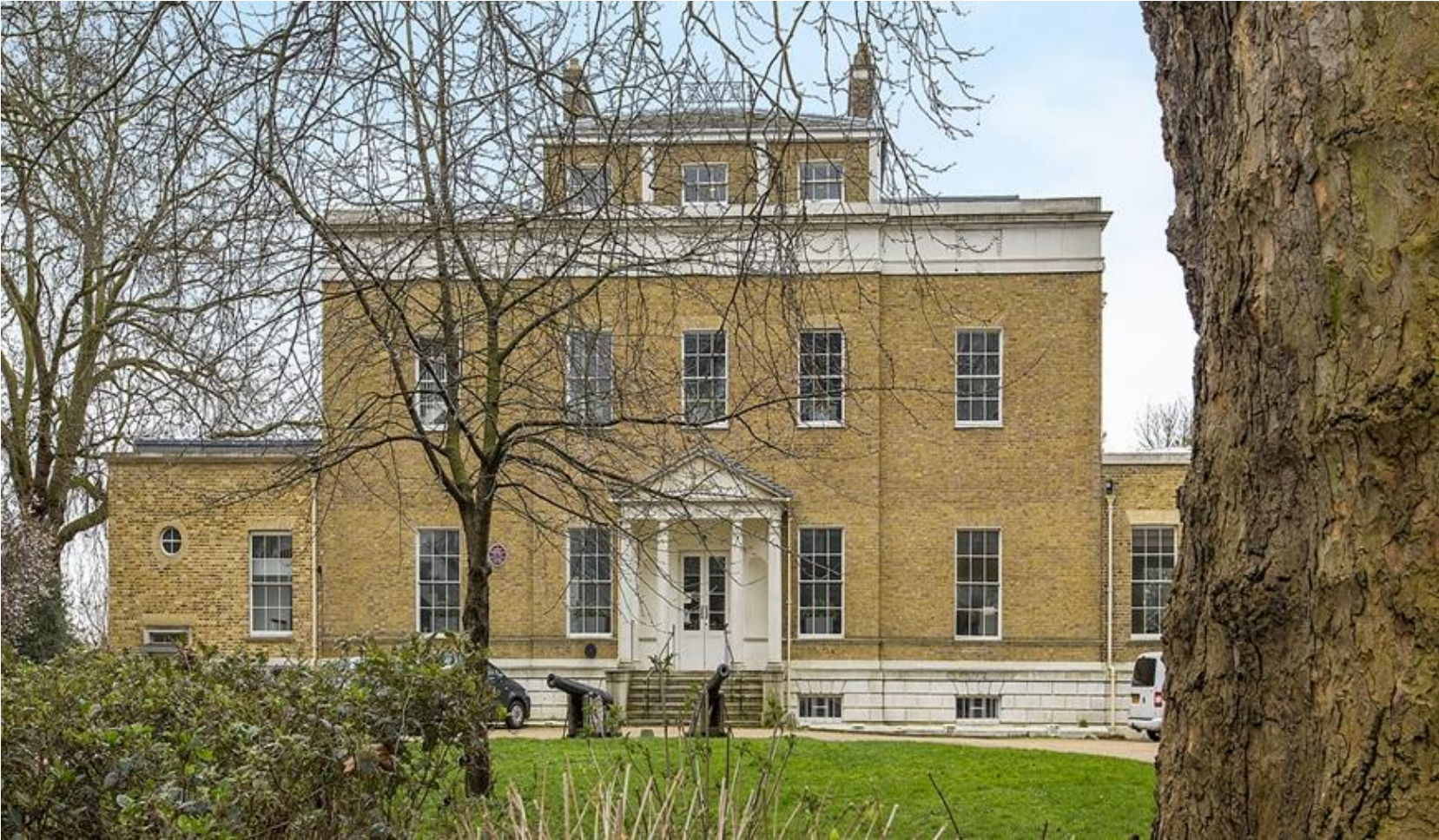
Grade II Listed Manor House, Old Road
