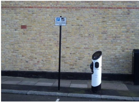
Electric car charging point, Kellerton Road
