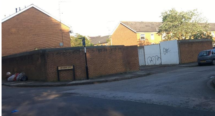
Garages, crn Osberton Road and Millbank Way, SA12
