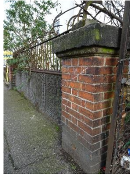
Bridge, Eastdown Park
