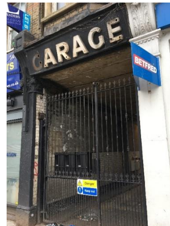
Old Garage Entrance, Lee High Road
