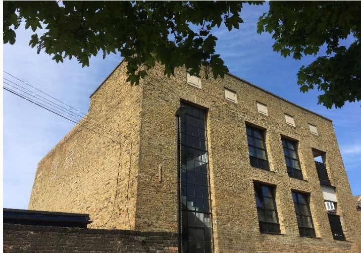
Depository and Auction House converted into flats, Old Road
