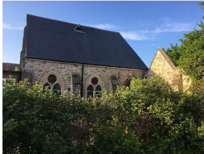
United Reformed Church, Burnt Ash Road
