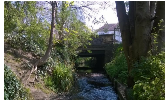
River Quaggy, Weigall Road bridge
