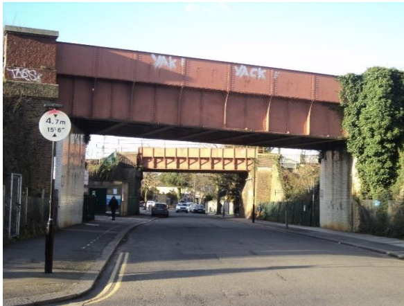
Two railway bridges at Manor Lane
