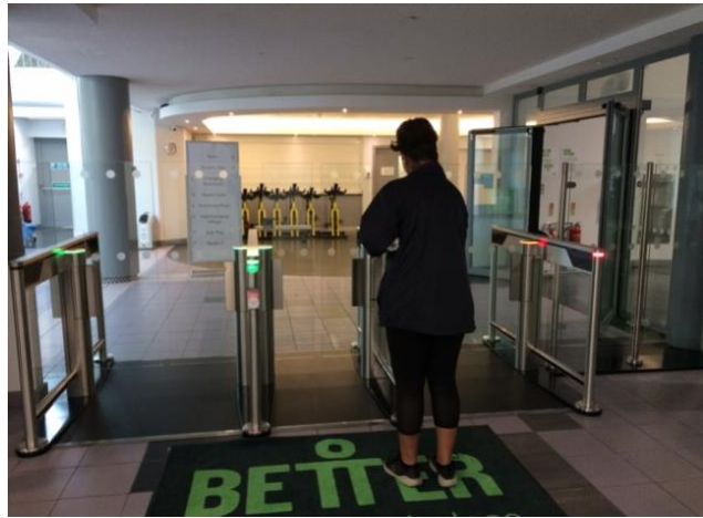
Image of access control turnstiles.
