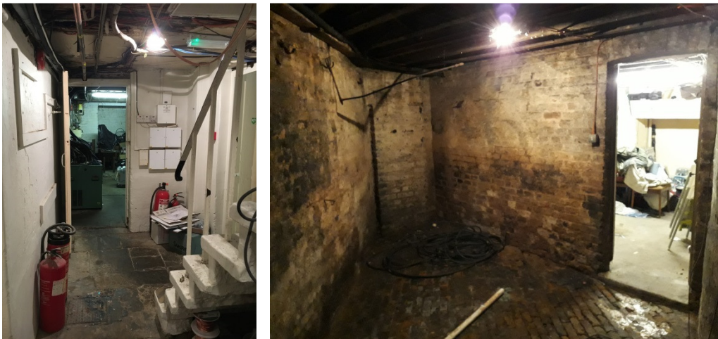
Figure 3.17 – Historic floor and wall surfaces are visible in places
