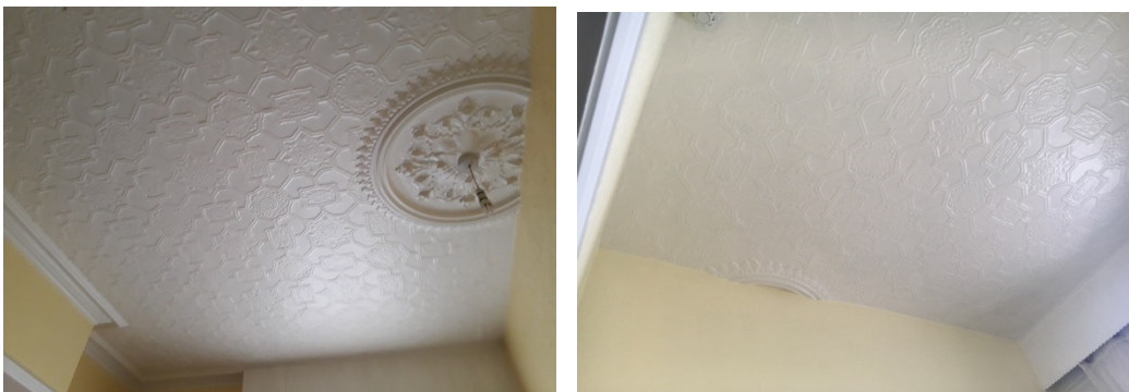
Figure 3.26 – Ceiling rose within Bedroom 2, split by a modern partition between Bedrooms 2 and 3.
