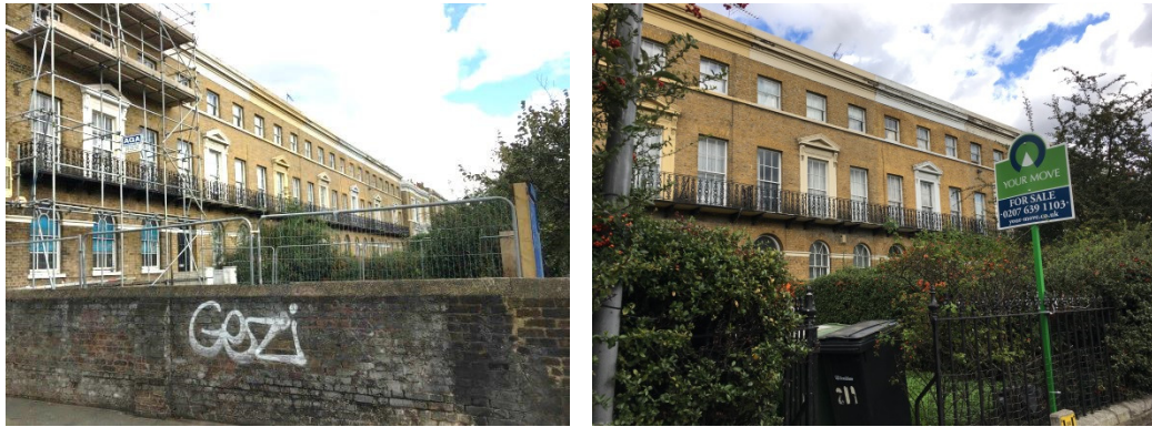
Figure 3.42 – Victorian townhouses front the north side of New Cross Road.
