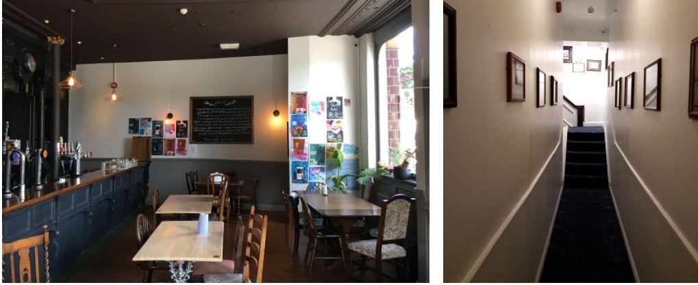
Figure 3.14 – Partitions have been inserted within the original pub space to create an access corridor to the hotel accommodation.
