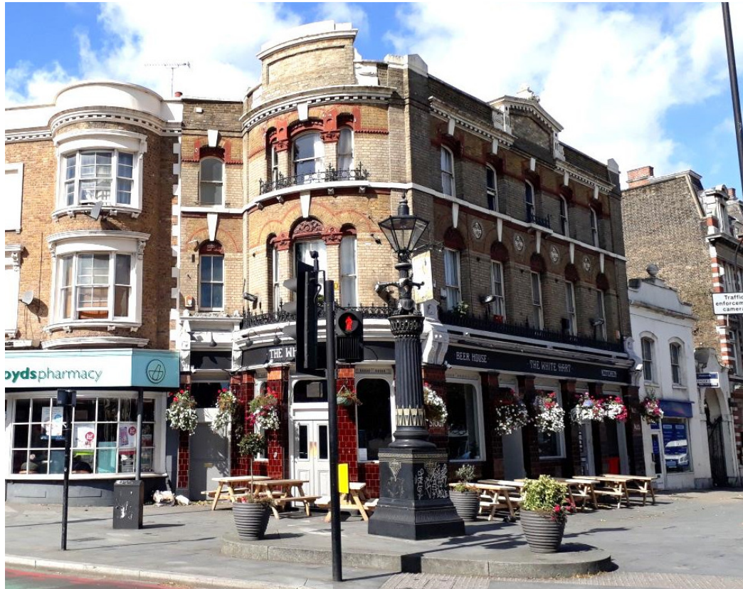
Figure 3.8 – The White Hart Public House, No.184 New Cross Road.
