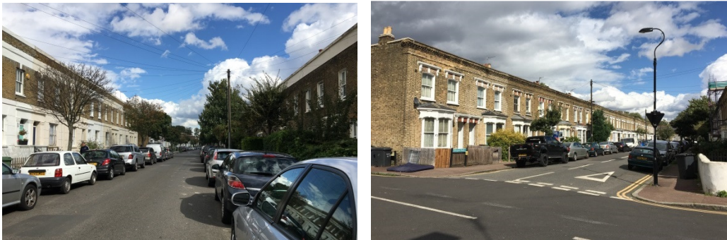
Figure 3.47– This part of the conservation area is characterised by domestic streets and modest terraced houses, and overall the atmosphere is much more calm and quiet than the frenetic nature of New Cross Road.
