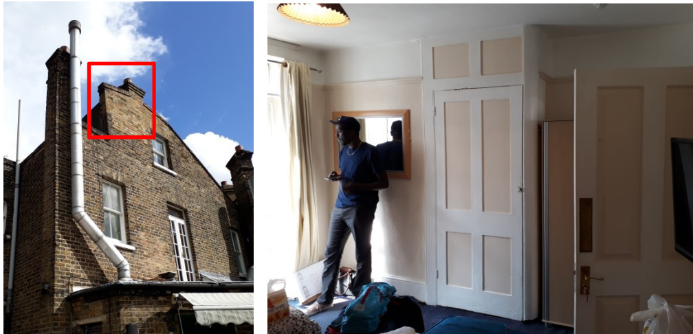
Figure 3.31 - Chimney corresponding to thick portion of wall within Bedroom 5.
