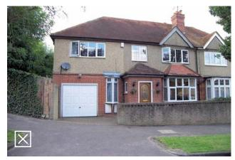
Fig 4.16: Unacceptable as it is not subordinate and the width is more than half of the existing building
