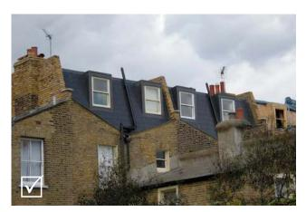
Fig 5.37: Acceptable -Butterfly form retained with slope of mansard running down to meet the existing eaves (please note that proposals should not include drainpipes)
