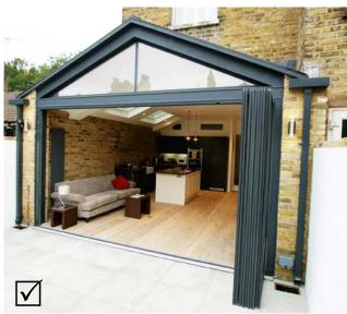
Fig 4.7: The extension distinguishes itself from the host building while retaining some traditional elements and has a positive relationship with neighbouring properties due to the restricted height on the boundaries
