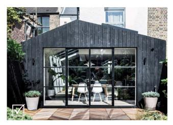
Fig 4.22: This wrap around extension pitches to achieve an appropriate height on boundary.
