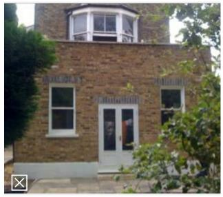
Fig 4.6: Unacceptable because the single storey rear extension is incongruous. This negatively impacts on the integrity of the original building form because it is too high, impacting on the first floor rear bay window
