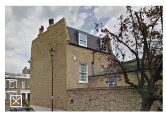
Fig 5.36: Unacceptable - Roof extension does not retain butterfly roof form
