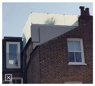
Fig 4.26: Visually intrusive balustrade detracts from the character of the building by reason of its siting close to the rear elevation.
