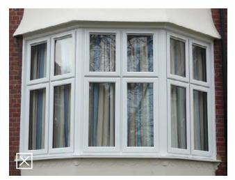
Fig 6.1: The replacement of traditional style windows on heritage properties with modern UPVC windows can be hugely detrimental to the properties' character
