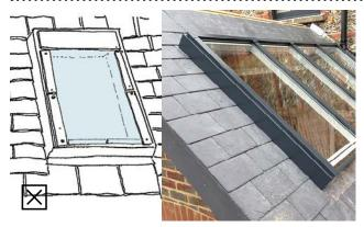
Fig 5.8: Unacceptable in conservation areas due to its protruding form
