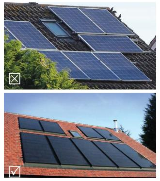
Fig 6.10: Solar panels should be placed symmetrically within the roof slope to minimise the effect on the external appearance of the building.
