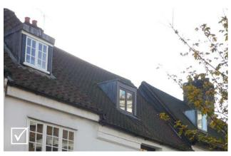
Fig 5.12: Acceptable example of dormer. They respect the proportions of the windows below and are an appropriate size
