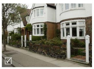
Fig 6.7: Existing original railings, gates and gateposts should be retained and refurbished
