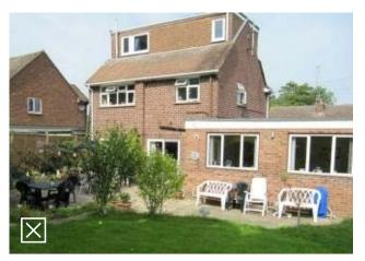
Fig 5.19: Unacceptable owing to the obtrusive nature of the extension. This obliterates the ridge, gable and sides
