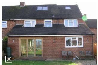
Fig 4.3: Unacceptable because the extension overwhelms the original dwelling and impacts on the first floor windows.
