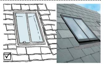
Fig 5.9: Rooflights in conservation areas should be small traditional 'conservation style' set flush within the roofslope
