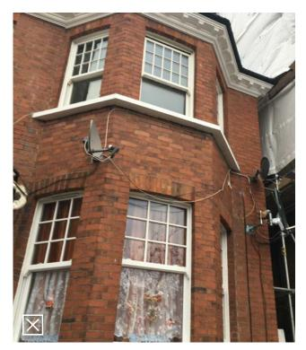
Fig 6.11: Satellite dishes should not be placed in front elevations.
