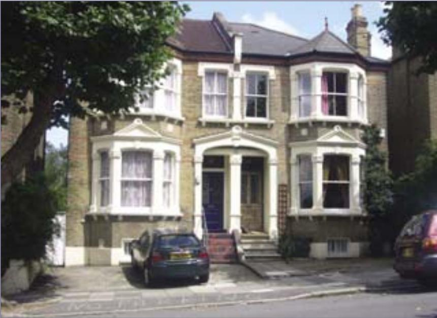
Roofs were originally covered with Welsh slates although in many instances natural slate has been replaced with ridged concrete tiles to the detriment of the house's appearance. A fishscale effect remains on many hipped bays. These should be preserved or replicated.
