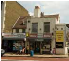
315-319: The 'M' shaped roof, Georgian paned windows and central chimney stack, clay-tile roof and small dormer are important features of this mid-18th-century pair of houses
