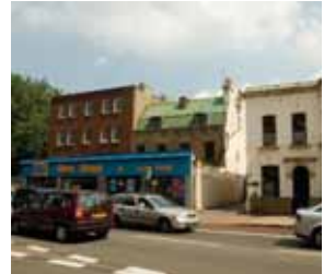
295-305 Lewisham High Street. The old houses would 'read' better if two separate shopfronts were reintroduced
