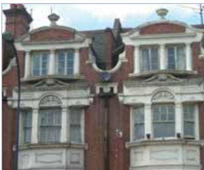
Detail at 318-320 Lewisham High Street
