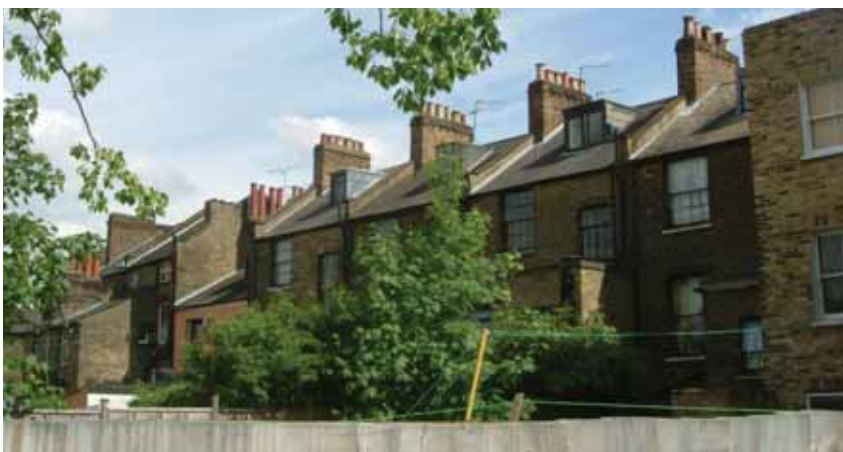
Rear elevations (Ladywell Road)
