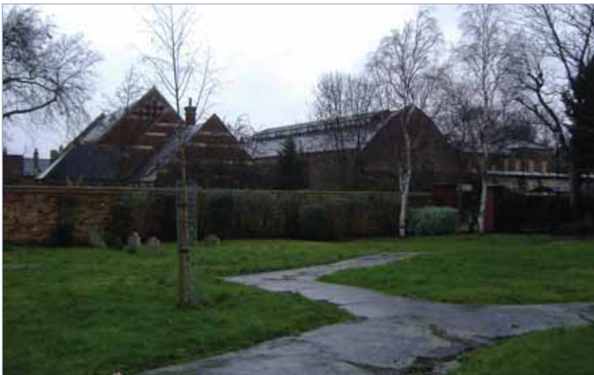
The rear of St Mary's Centre and former Ladywell Baths (Playtower) seen from the churchyard
