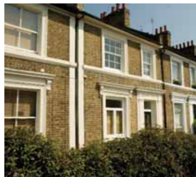
Yellow stock brick with stucco dressings on terrace houses
