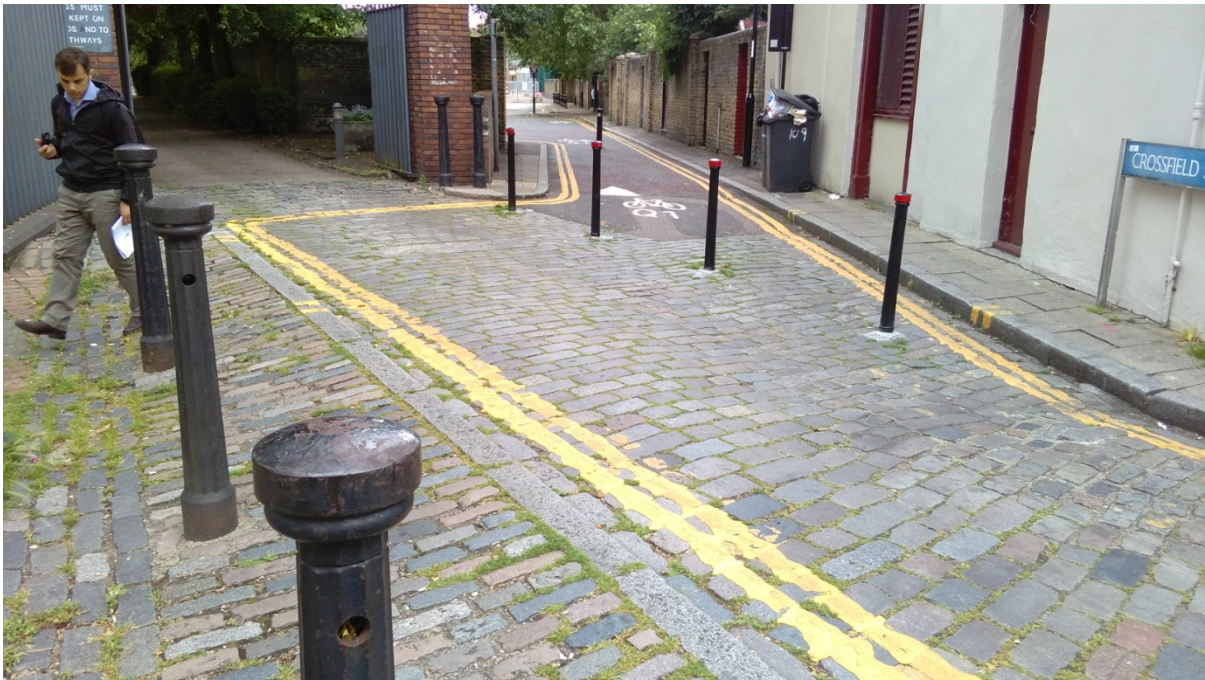
Plate 5. View of Crossfield St. Level difference clear at bollard line. Quietway closure motorised traffic visible centre rear.
