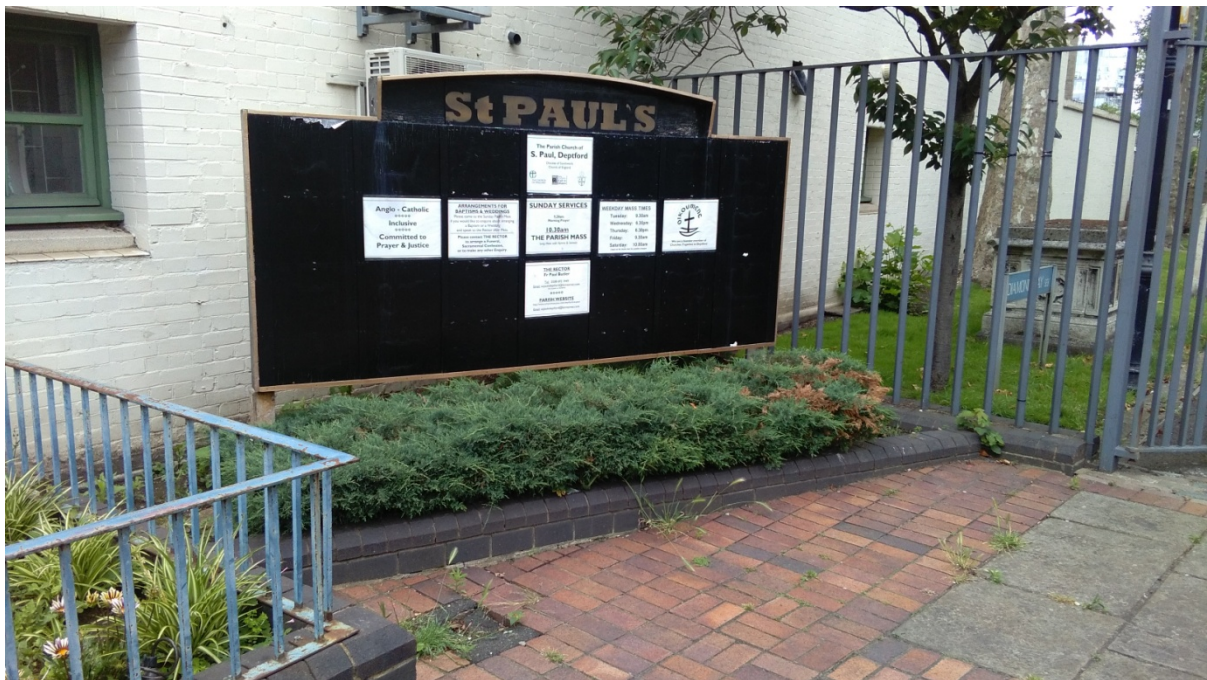
Plate 6. View of notice board of be replaced and detail of iron railings and engineering brick walls
