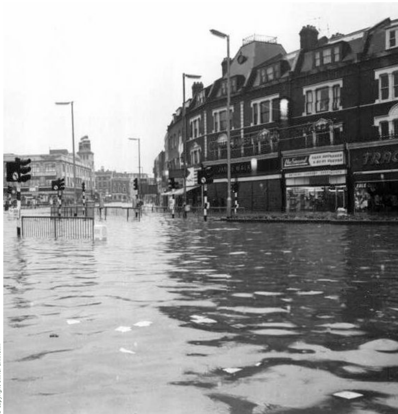
Lewisham Town Centre during flooding in 1968.
