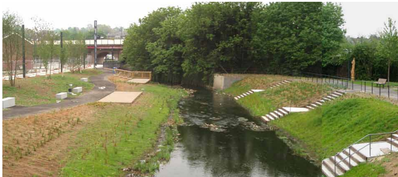
Immediately after restoration
