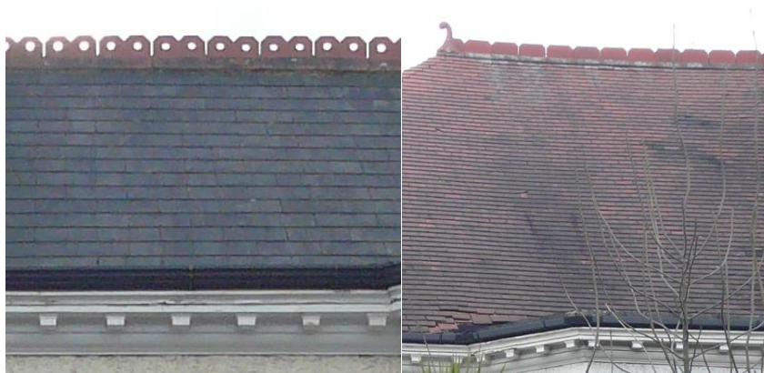
Images 42 and 43: Welsh slate is the historic roof covering material in Gaynesford Road (left) and red clay tile is the historic roof covering material in Perry Vale (right).
