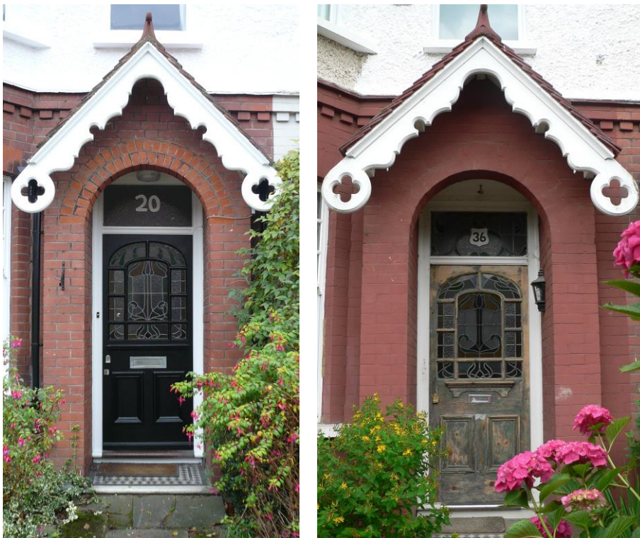
Images 51 and 52: The Christmas houses feature a red brick porch with the door beneath a round arch, the pitched roof (topped with ridge tiles ending in a finial) is detailed at eaves level with cinquefoil (four leaf clover) piercing on the barge boards. The cinquefoil piercing is a Christmas trademark, found on houses built by him around this time elsewhere in the borough.
