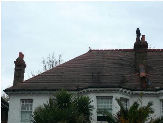
Images 69 and 70: Replacement of roof covering with non-traditional materials can detract from the appearance of the property
