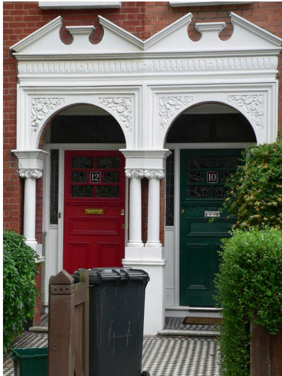
Image 2: Numbers 10 and 12 Gaynesford Road, recessed porches with elaborate stucco surrounds.
