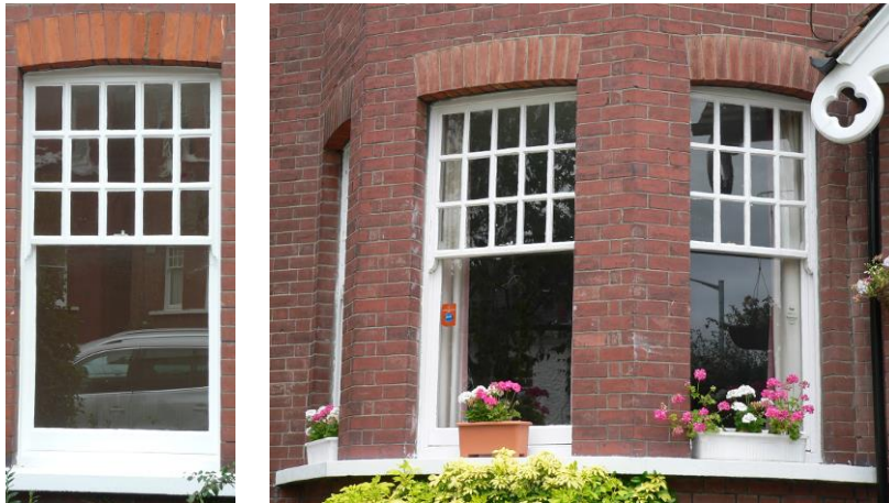
Image 47 and 48: Queen Anne style windows, a single window (left) and a bay window (right).
