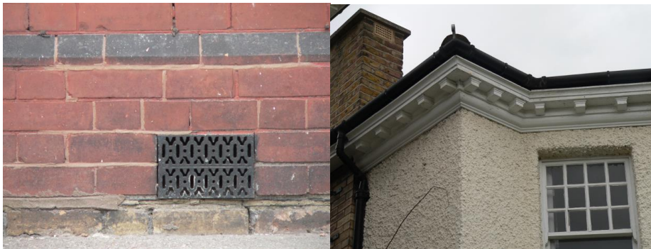
Image 40: Red brick laid in Flemish bond is the usual walling material.
