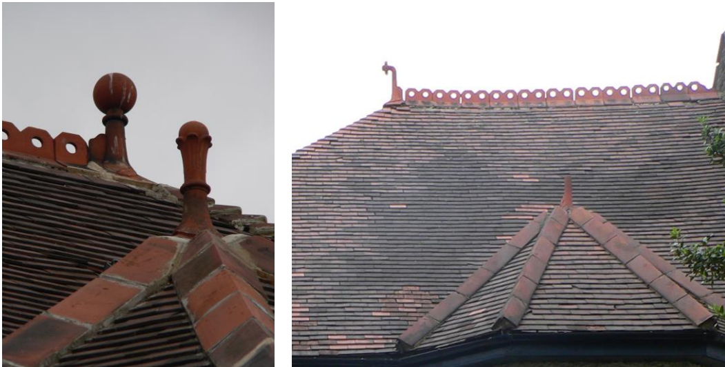
Images 55 and 56: Terminations are marked by finial tiles in ball or hook designs.
