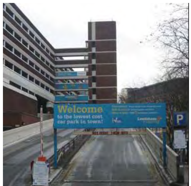
Existing town centre multi-storey parking
