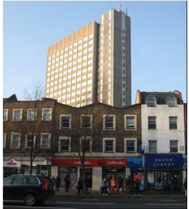
Tall buildings and surroundings
