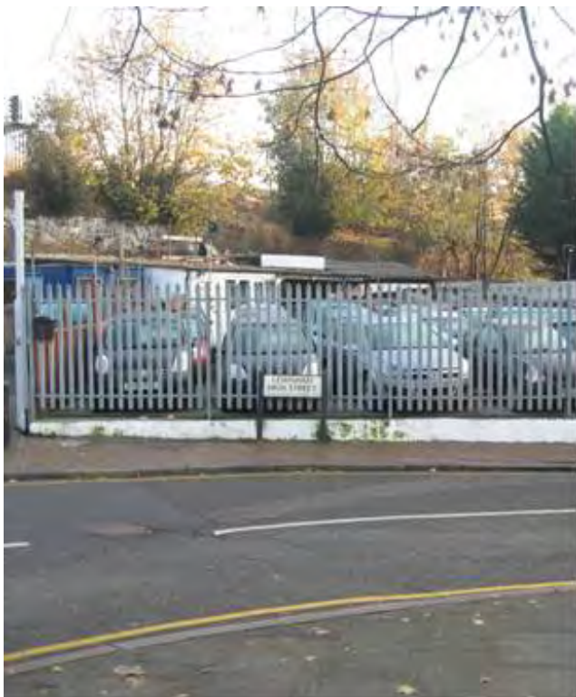
Kings Hall Mews site with railway embankment
