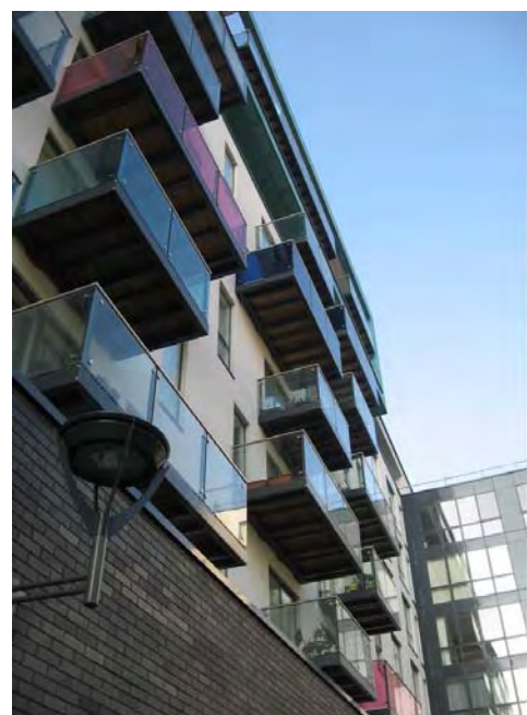
Completed development: Conington Road
