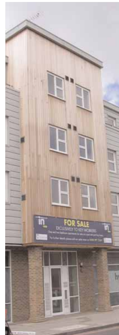
Keyworker housing, Lee High Road
