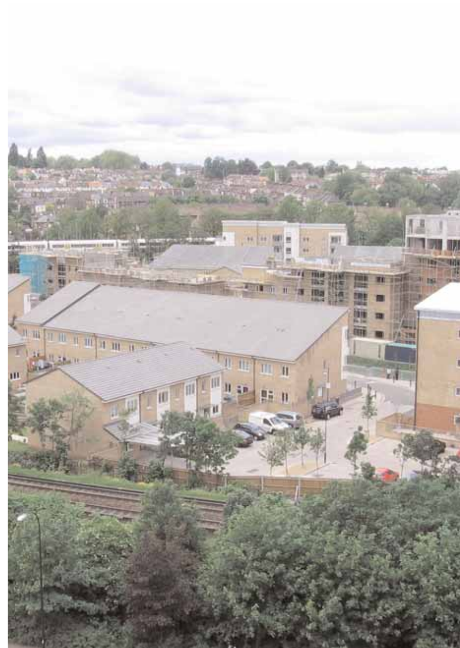
Sundermead Estate undergoing redevelopment
