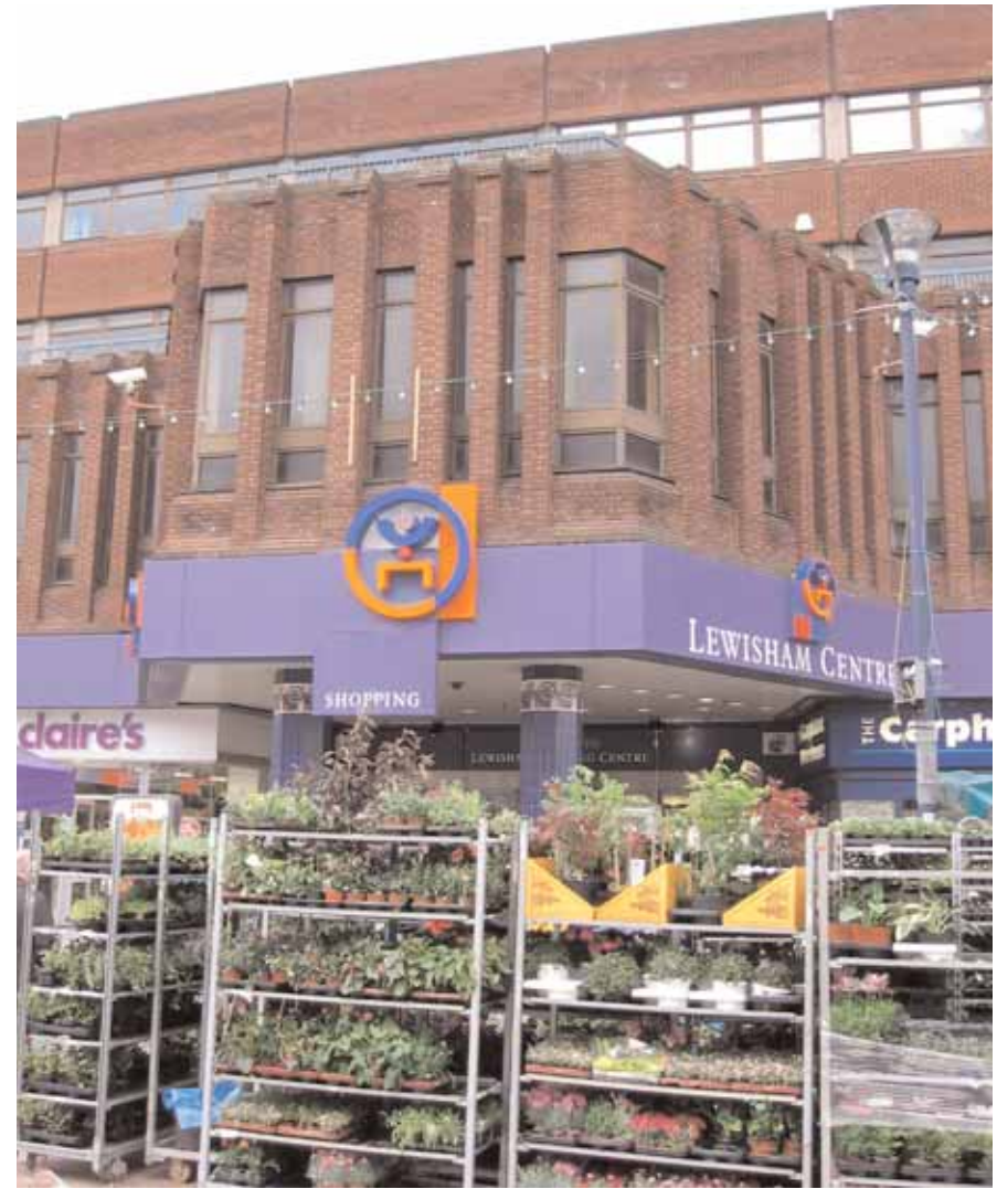
Lewisham Centre and the street market, the heart of the town centre
