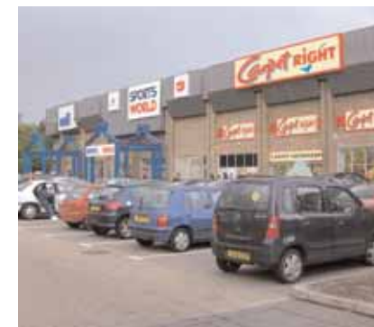
Thurston Road retail frontage.
