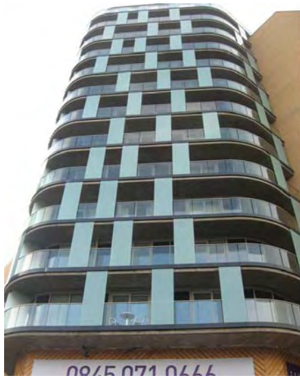
Development south of Loampit Vale
