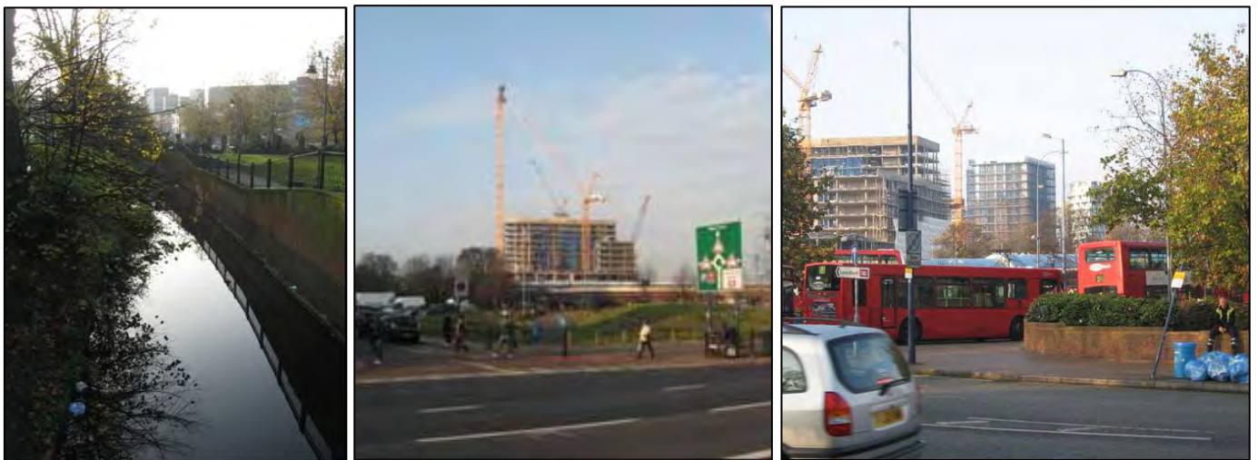
Lewisham Gateway site
