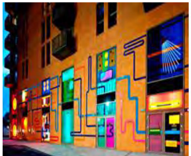
Loampit Vale energy centre
