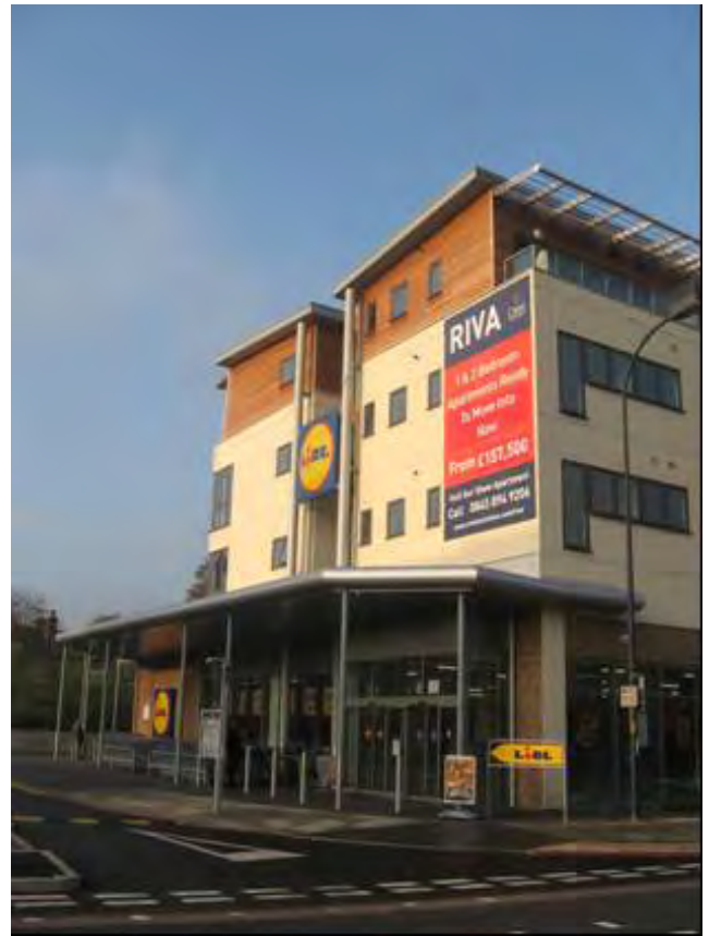
Completed development in Lee High Road
