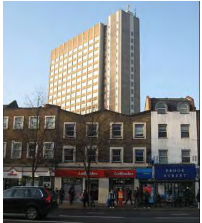
Tall buildings and surroundings
