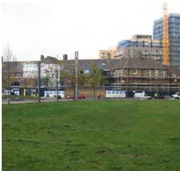
Redevelopment of Lewisham Bridge into Prendergast Vale through-school
