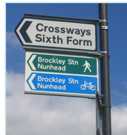
Signs neatly grouped on one pole.
