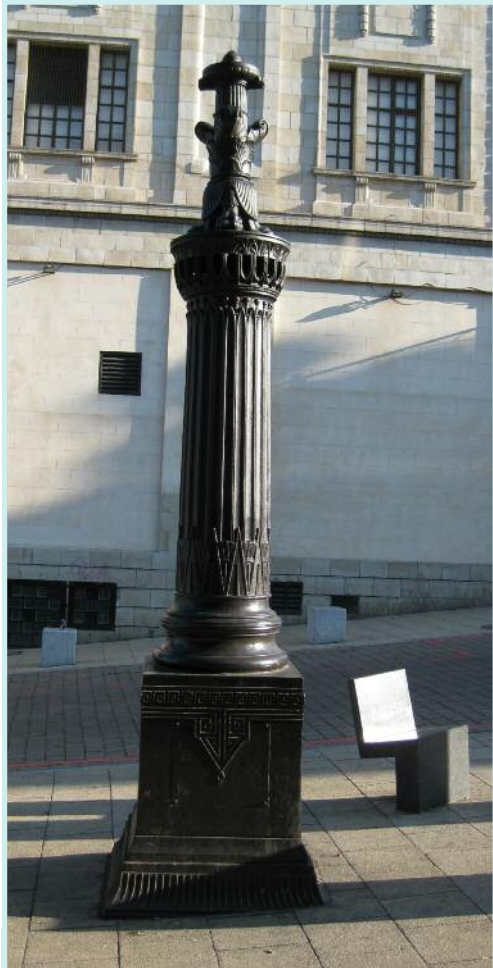
Decorative vent pipe in New Cross.
