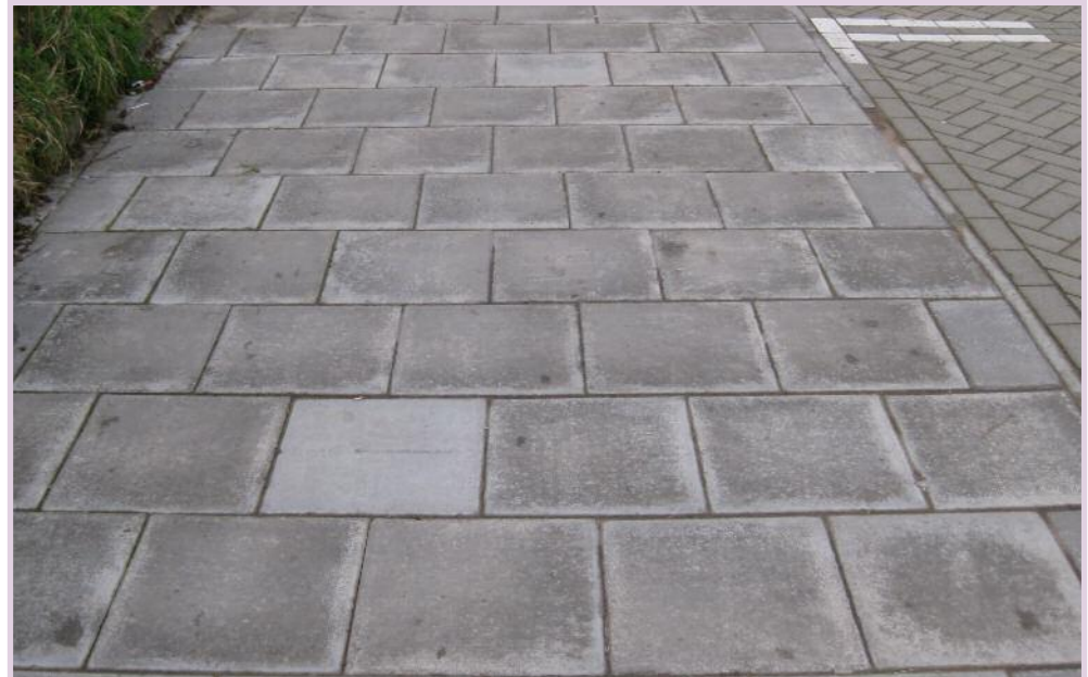
Block paving is stronger than concrete paving and therefore a good option when over-running vehicles might otherwise damage the footway.
