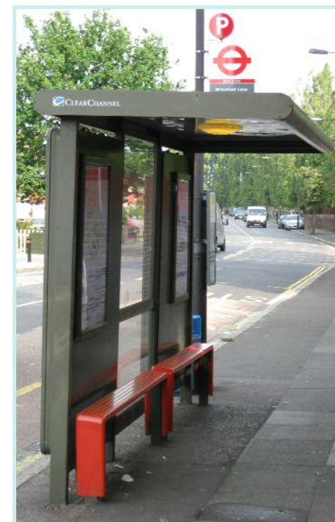
A cantilever bus shelter is a good option on narrow footways.
