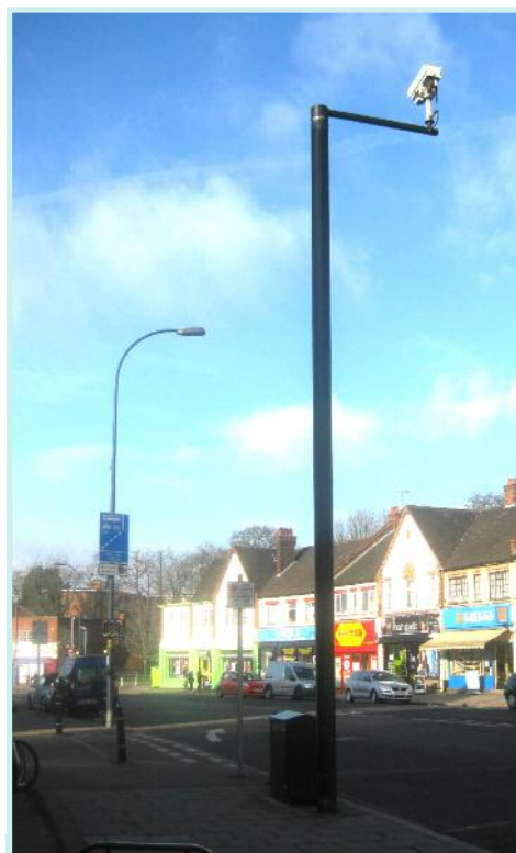
Narrower flange mounted tubular pole.
