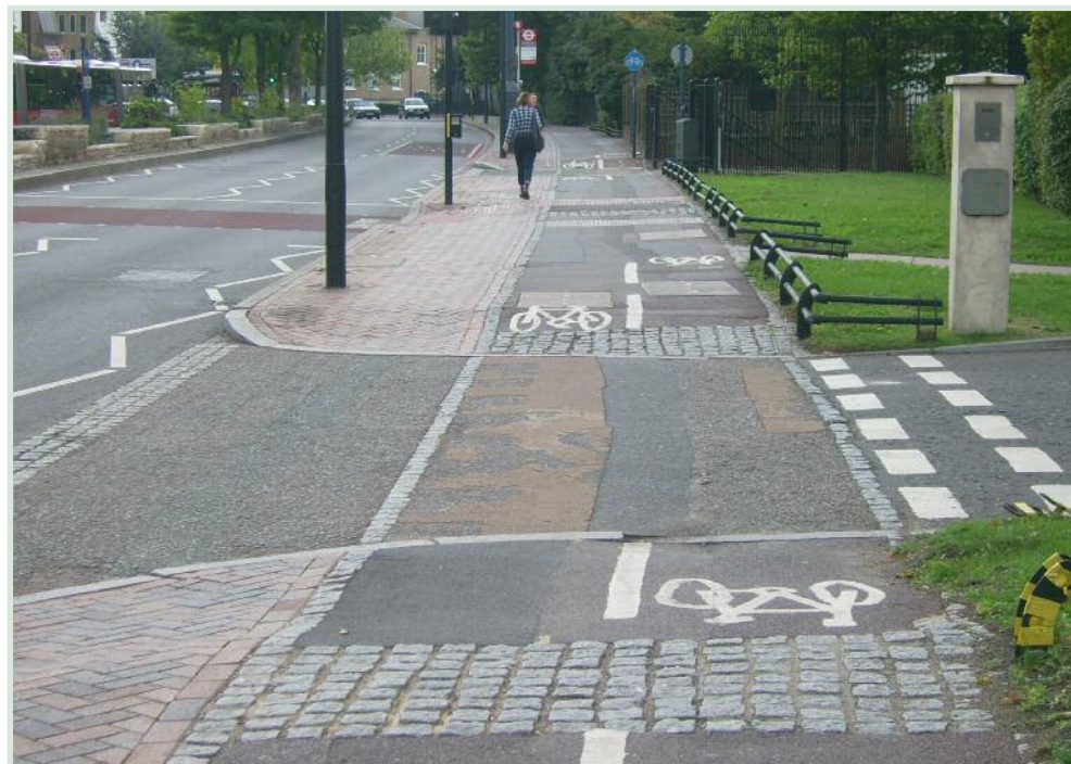
Anyone marking roads in Lewisham must comply with Traffic Signs Regulations and General Directions 2002. Cycle markings are used to indicate a cycle route or other facilities for cyclists.
