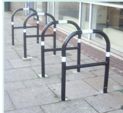
The 'Hammersmith' cycle rack is functional and simple, and includes a reflective strip so it can be easily seen in low light.
