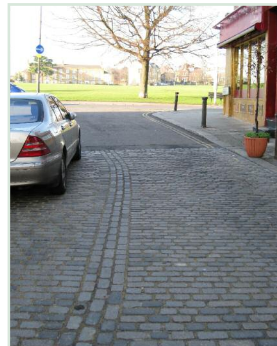
Granite setts, such as these in Blackheath, should only be used where there are low volumes of traffic.
