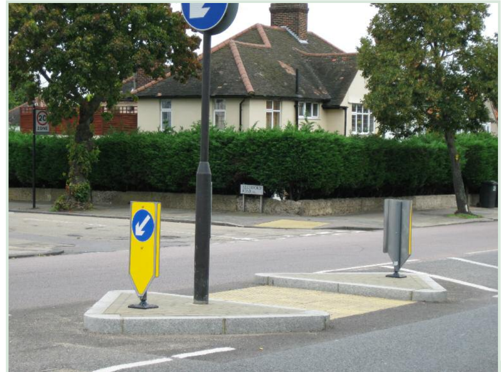
Pedestrian refuges are generally to be found on wider roads with relatively low levels of traffic.
