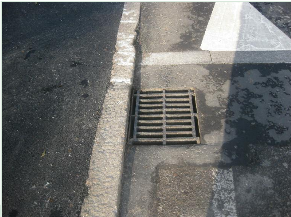
Gully cover on the carriageway.
