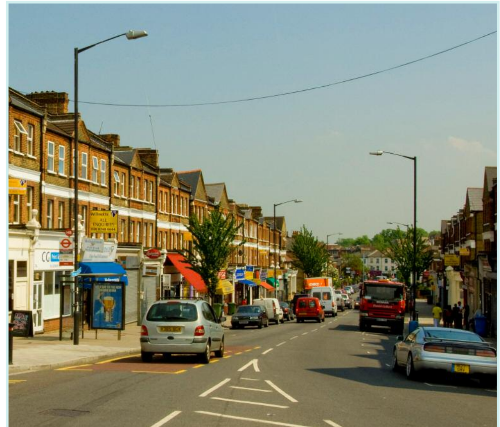
From July 2011, Skanska-Laing will take on responsibility for the design, build, maintenance and operation of Lewisham's lighting columns for a period of 25 years.
