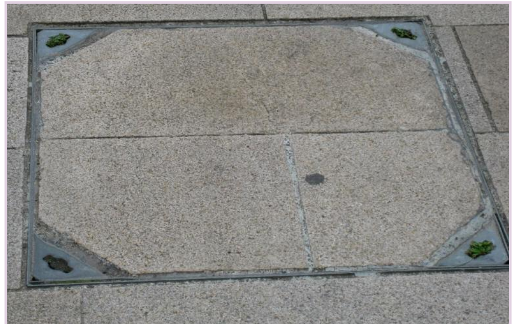
The lines of surrounded paving slabs continue within an inset inspection cover to create an appearance of continuity.
