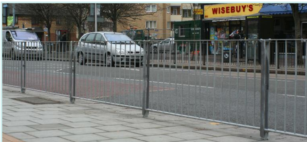
Guardrails add to street clutter and should be avoided on the footway unless a safety audit recommends otherwise.
