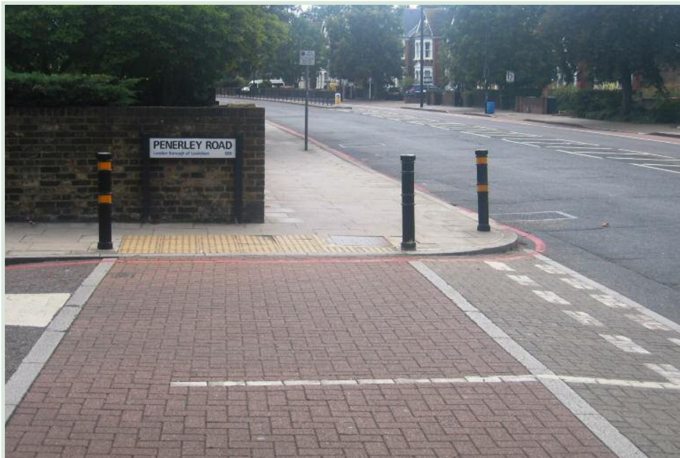
A raised entry at the junction of a main road and side road will encourage vehicles to slow down as they turn into the quieter street
