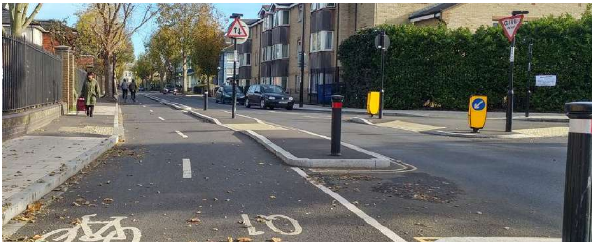
Figure 15 – recently completed Quietway 1
