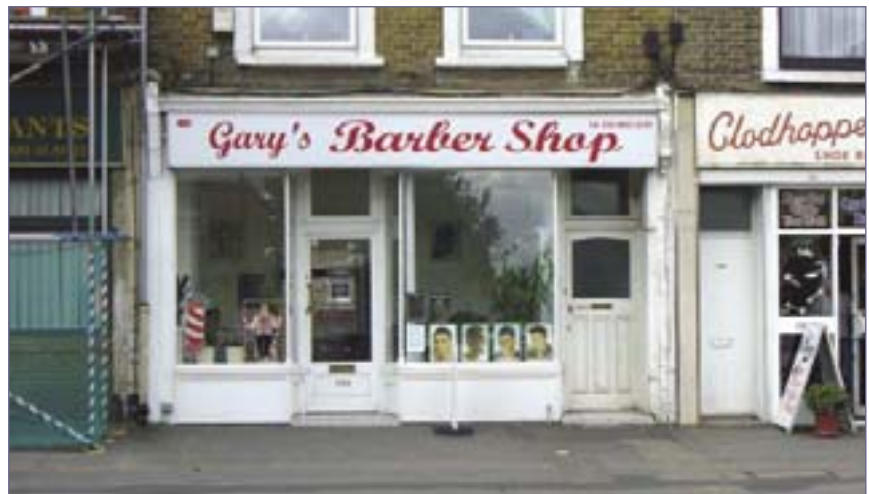
Original shop front with modern fascia
