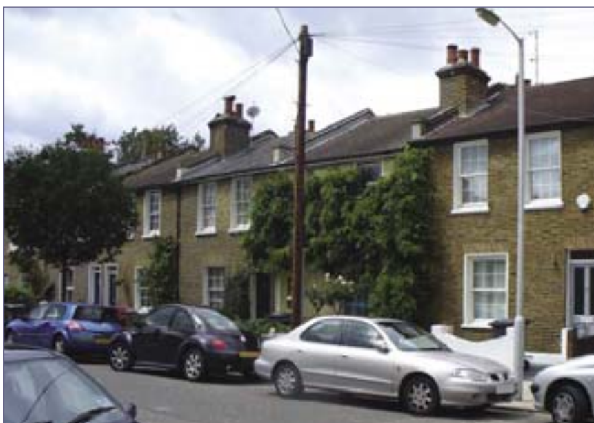
Early terraced housing on Brightfield Road, note the original six over six paned sash windows.
