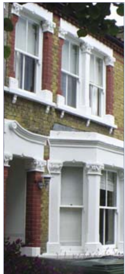
Details of doors and sash windows
