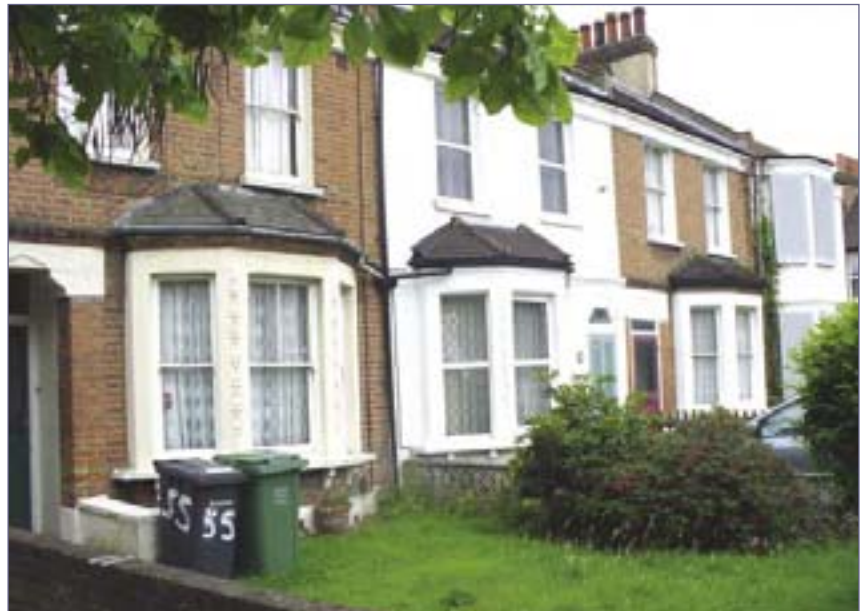
Lampmead Road (south side), incised foliage motifs around windows and doors
