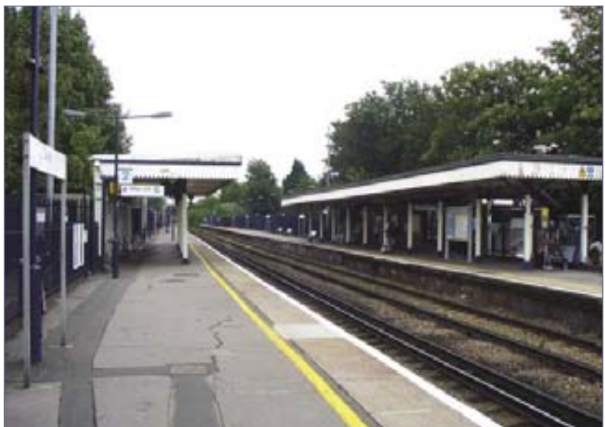
Platform shelters at Lee Station
