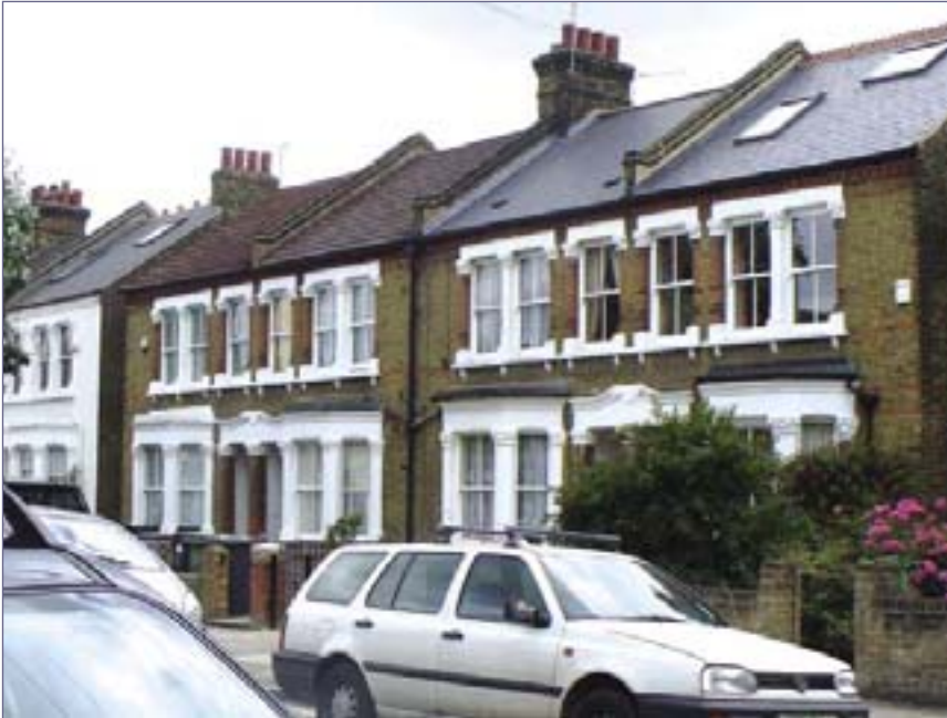
View along north side of Effingham Road with repeated architectural detailing
