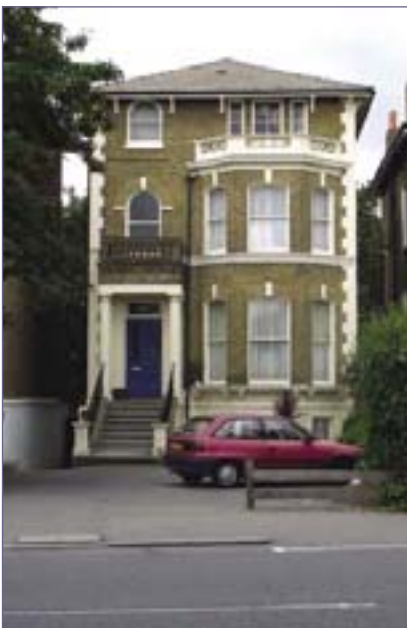
Burnt Ash Road: three-storey town house
