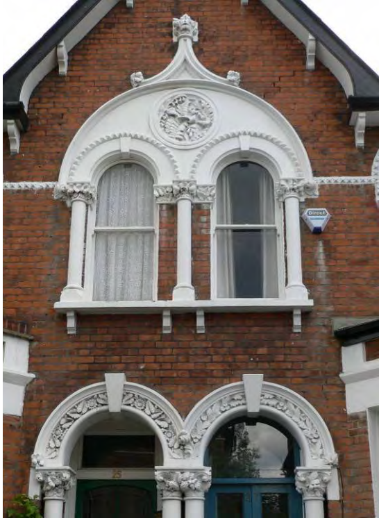
The round central stucco tympanum on red brick is one of the most elaborate features of the Jerrard properties.
