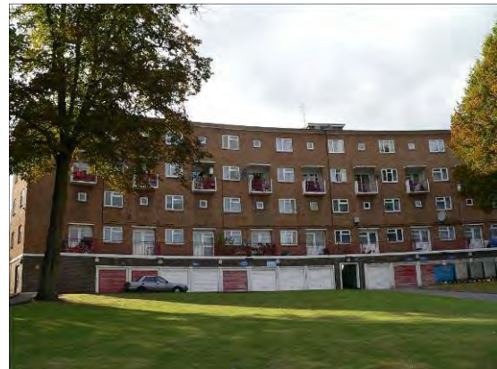
93-131 Ermine Road as seen from the Embleton Road.
