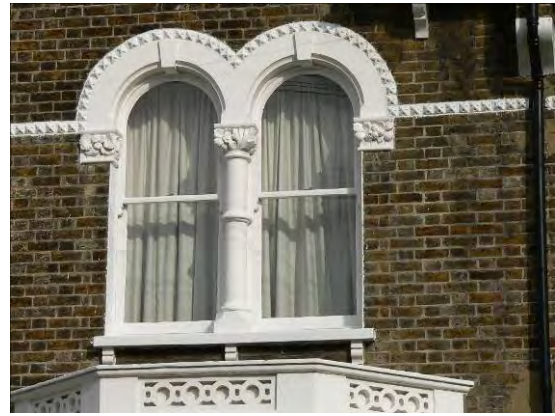
Decorative features to the properties include foliage capitals nail-head strings and strapwork parapets.
