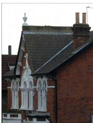
Roofscape detail – gable topped with finial.
