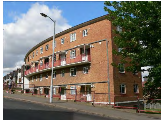
93-131 Ermine Road as seen from the south-west.
