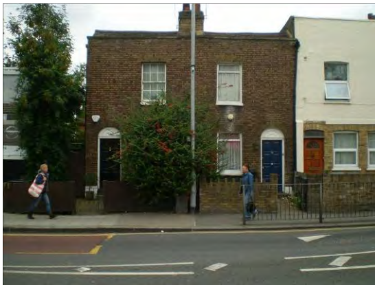
Early 19 th century dwellings in Ladywell Road (south-side).
