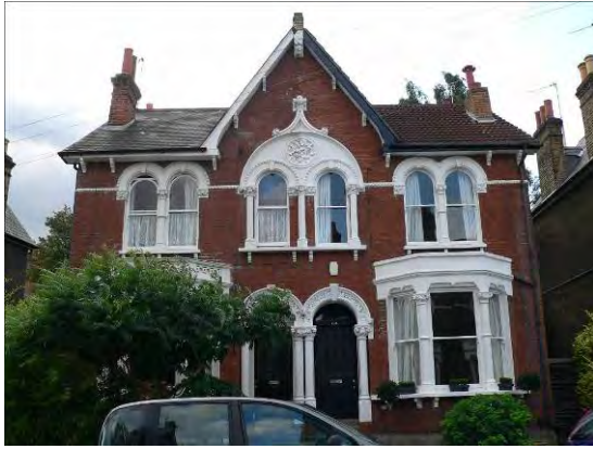
The semi with central outward-facing gable is the most attractive type of Jerrard's buildings thanks to the stucco tympanum that surrounds the central windows on the upper floor level.
