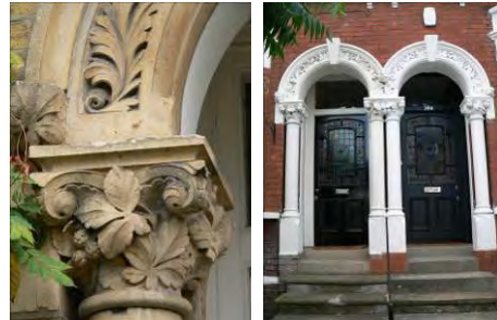
Window and door surrounds and columns are made of stone and terracotta, although these have now mostly been painted.
