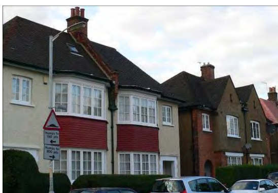
Above: Render, brickwork, and hipped plain tiles roof
