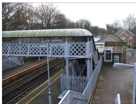
The lattice-girder footbridge of Ladywell Station.
