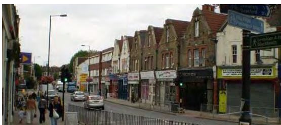
Commercial Development (Ladywell Road, north-side).
