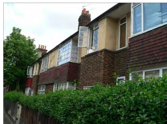
Johns Court at the western end of Gillian Street.
