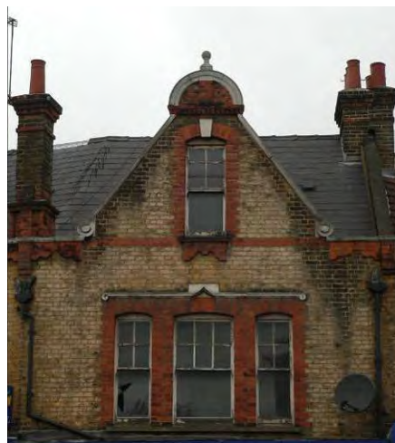
Red brick is subtly used to highlight features such as window surrounds, banding, eaves details and the shaped gable at 'The Pavement'.
