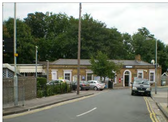
The Ladywell Railway Station as seen from Ladywell Road.
