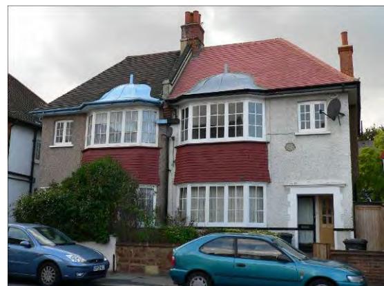
Early 20 th century semi at Algernon Road with wide, full-height canted bays topped with bell-shaped canopies.
