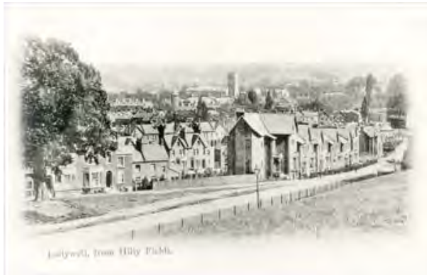
Views down Vicars Hill at the junction with Ermine Road, c.1899
