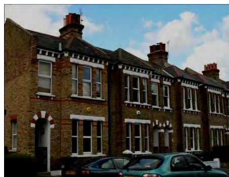
Polychromatic brickwork at the terraces in Gillian Street.
