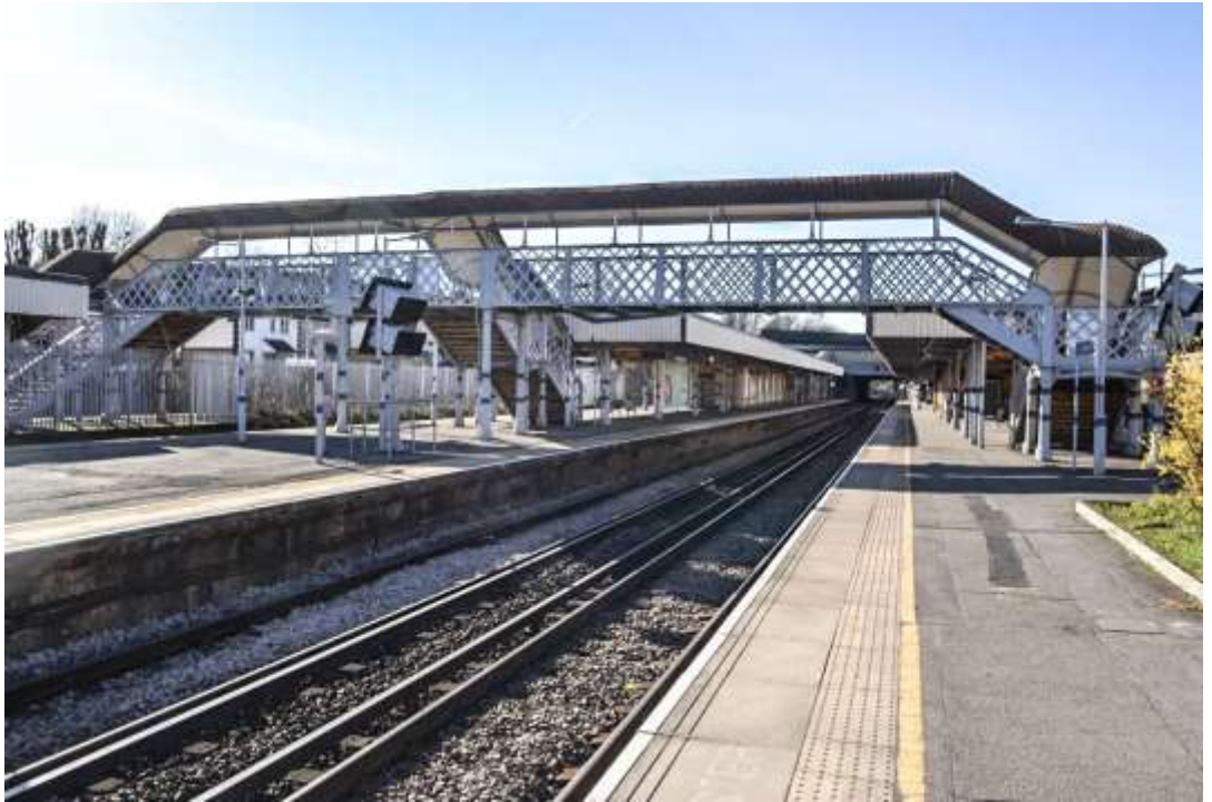
GROVE PARK STATION'S IRON FOOTBRIDGE WITH DECORATIVE SUPPORTIVE COLUMNS AND TRADITIONAL LATTICE DETAIL -"A WELL PRESERVED EXAMPLE OF ITS TYPE WITH THE STAMP AND DATE OF W. RICHARDS AND SON 1902." (SAVE BRITAIN'S HERITAGE). APRIL 2013
