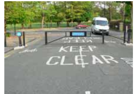
Fig.8.7 Modal filter: allows cycles through but not motors.
