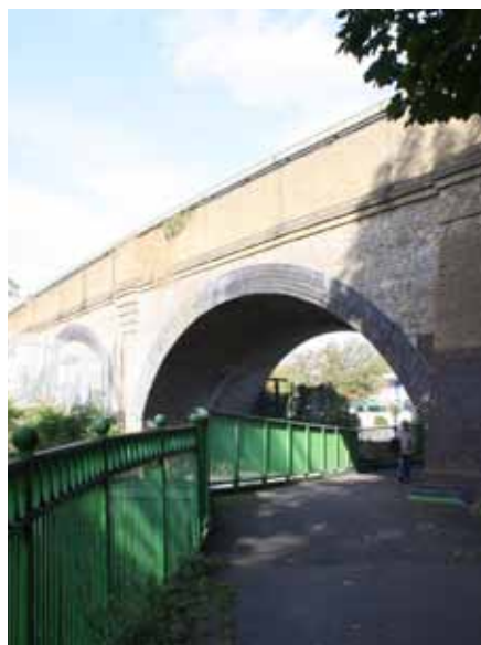
Pedestrian Link Under Viaduct
