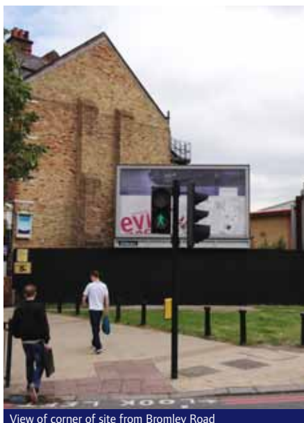
View of corner of site from Bromley Road
