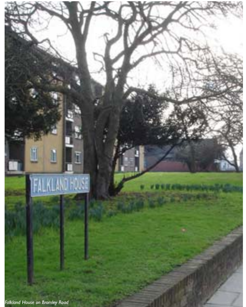
Falkland House on Bromley Road
