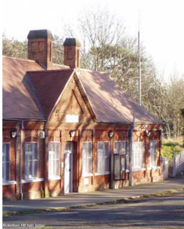
Beckenham Hill train station
