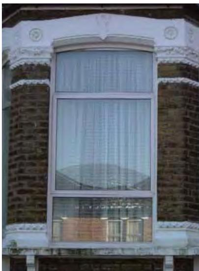
This aluminium window is unsuitable both in its materials and its design
