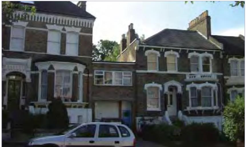
Two examples of side extensions which both close the gap between houses and alter the balance of the streetscape
