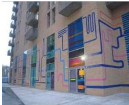
Renaissance Energy Centre Loampit Vale
