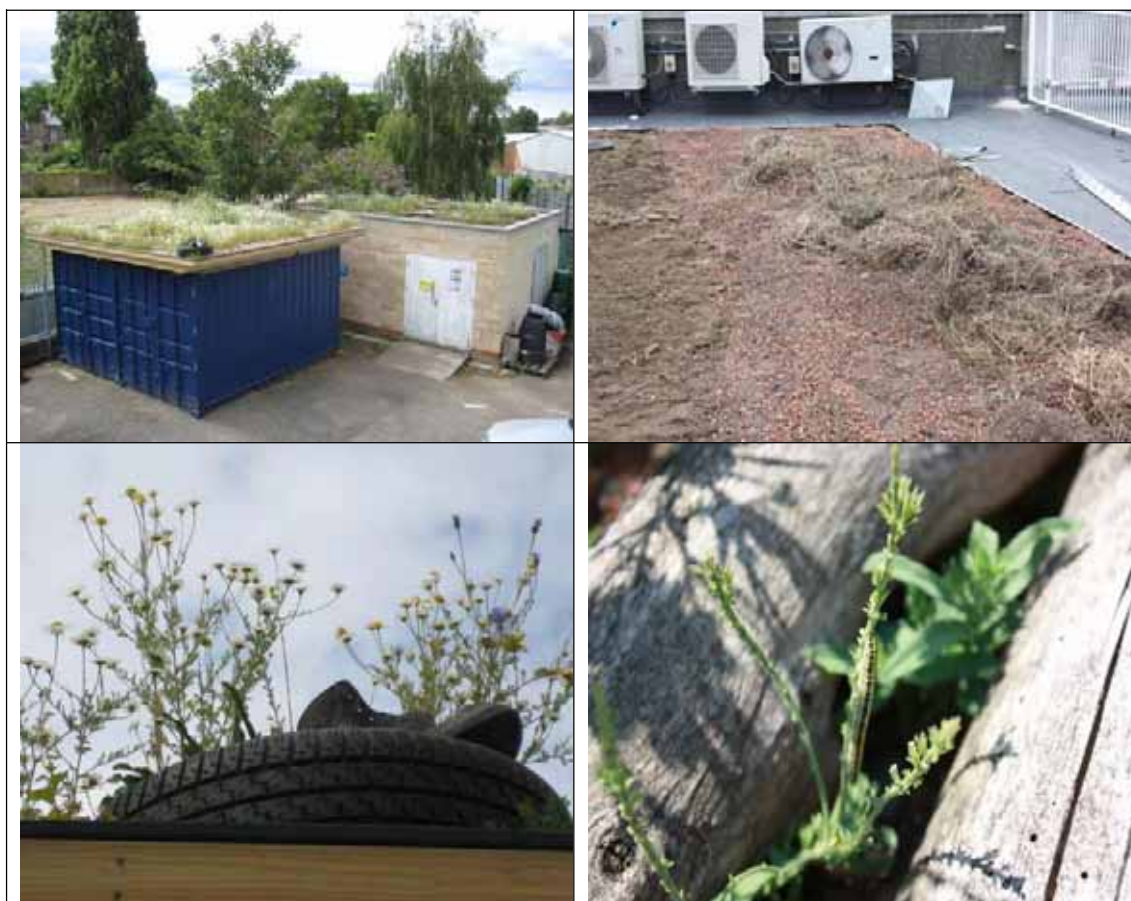
Figure 5.3: Living roofs in Wearside Service Centre
