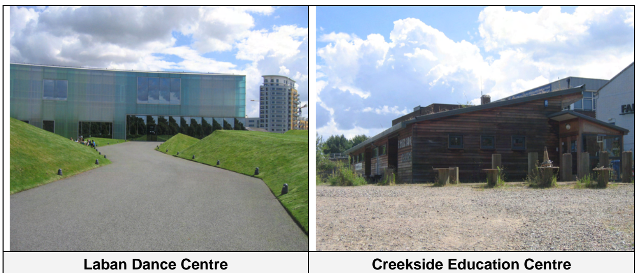
Figure 35: Living Roofs in Lewisham
