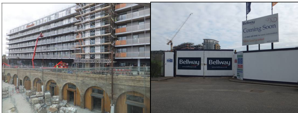
Photo 3.3: Kent Wharf construction site
