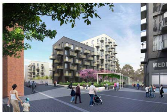
View of The Grove
