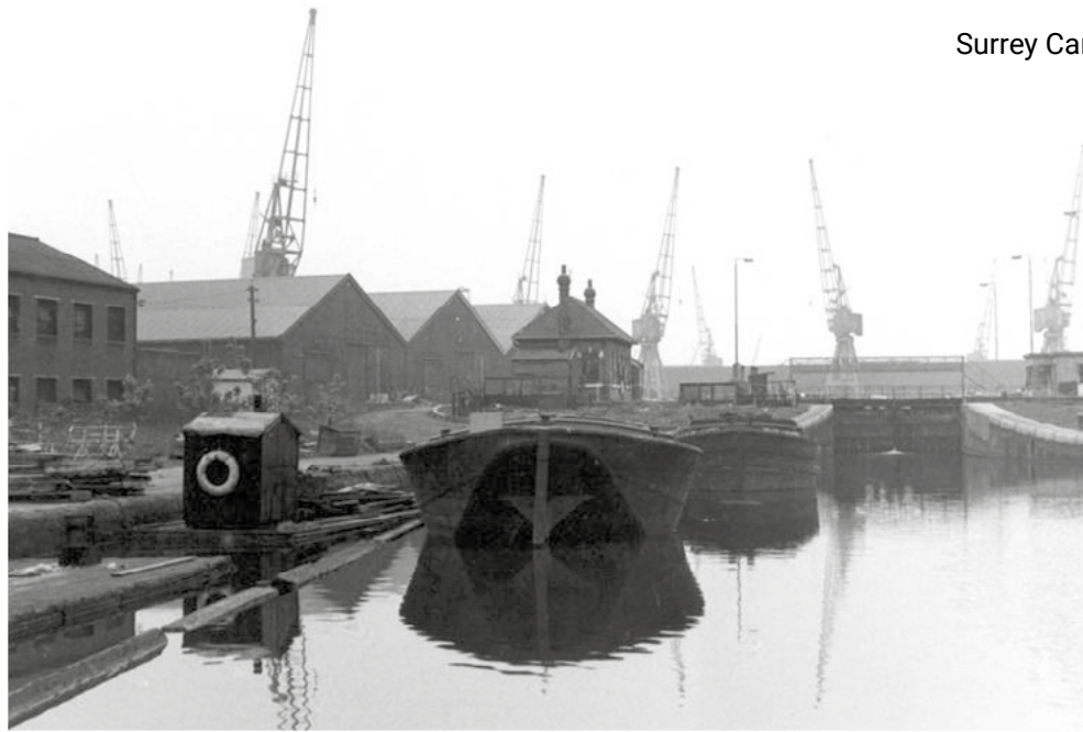
Fig.11 Timber Wharf in Operation (1970's)
