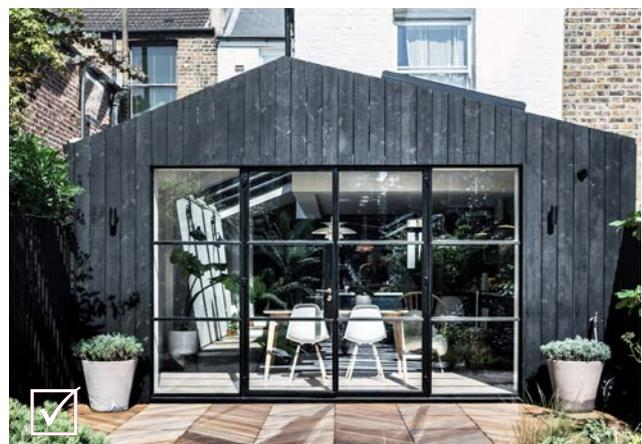
Fig 4.22: This wrap around extension pitches to achieve an appropriate height on boundary.
