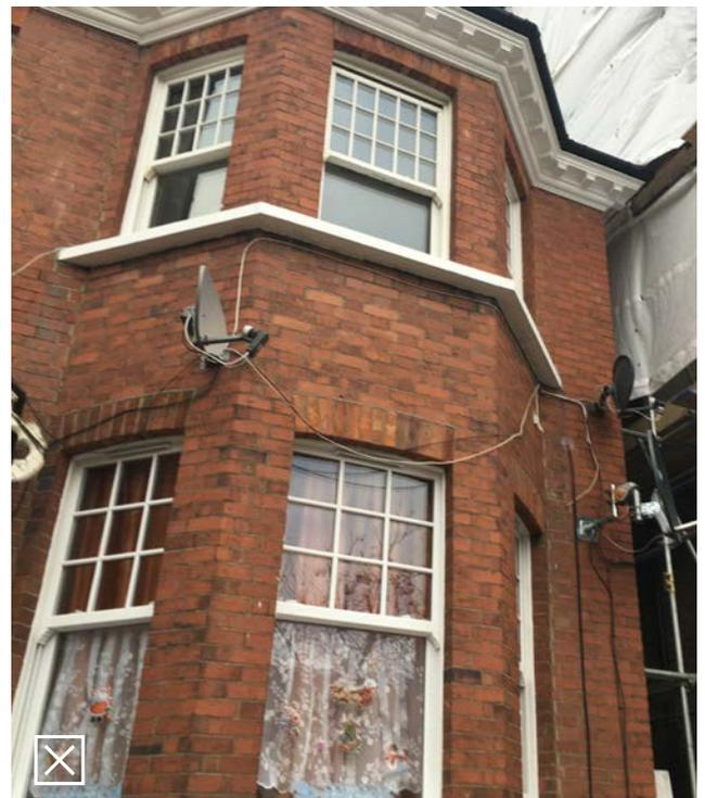
**Fig 6.11:** Satellite dishes should not be placed in front elevations.
