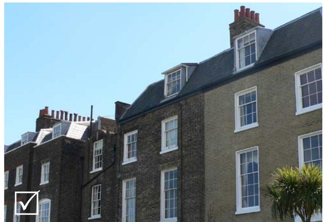
**Fig 5.11: Acceptable due to its slender, subordinate form and alignment with the elevation below**
