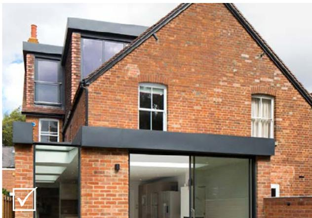
Fig 5.28: Acceptable due to sympathetic materials and they are both set in from the original roofline
