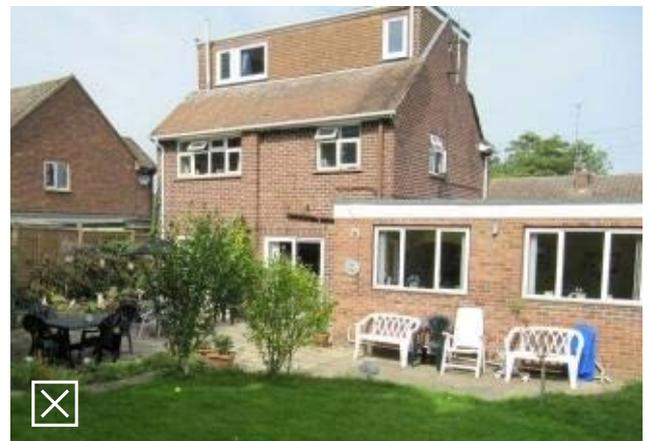
**Fig 5.19: Unacceptable owing to the obtrusive nature of the extension. This obliterates the ridge, gable and sides**
