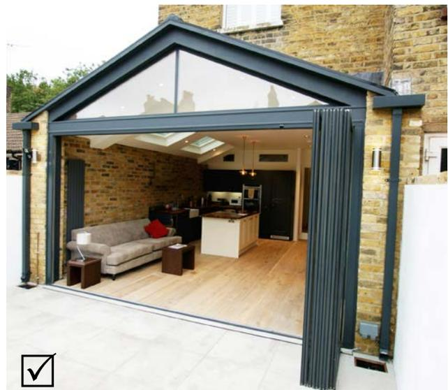
**Fig 4.7: The extension distinguishes itself from the host building while retaining some traditional elements and has a positive relationship with neighbouring properties due to the restricted height on the boundaries**
