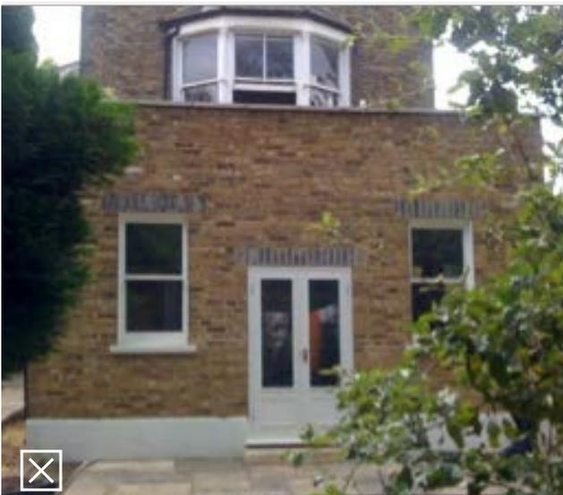
**Fig 4.6: Unacceptable because the single storey rear extension is incongruous. This negatively impacts on the integrity of the original building form because it is too high, impacting on the first floor rear bay window**
