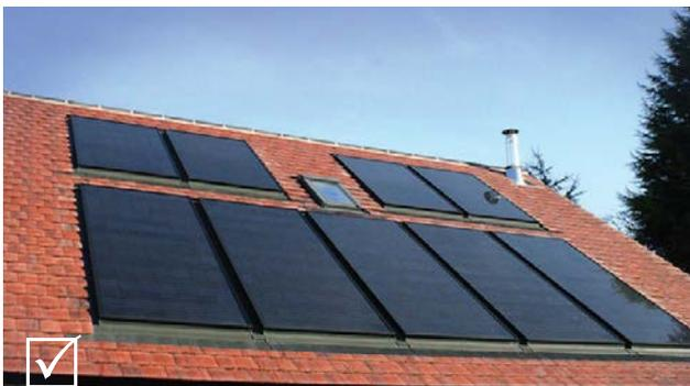
**Fig 6.10:** Solar panels should be placed symmetrically within the roof slope to minimise the effect on the external appearance of the building.
