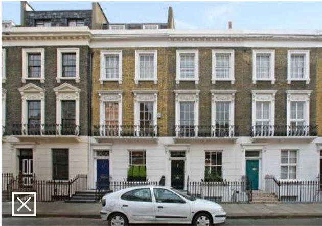
**Fig 5.33: Unacceptable mansard extension shown from front. Different proportions and heights result in incongruous roof form and lack of symmetry**
