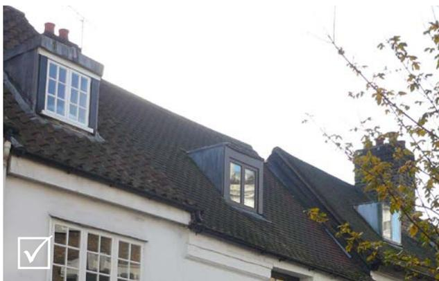
**Fig 5.12: Acceptable example of dormer. They respect the proportions of the windows below and are an appropriate size**
