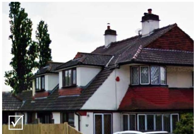
**Fig 5.21: Acceptable as the side dormers are subordinate to the roof and set in from all directions**
