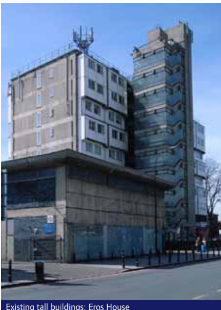
Existing tall buildings: Eros House
