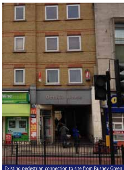
Existing pedestrian connection to site from Rushey Green
