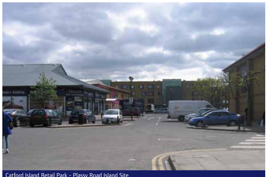
Catford Island Retail Park - Plassy Road Island Site
