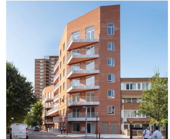
Fig. 4 Prominent corner design at Marklake Court, Weston Street, Kipling Estate, London SE1 3RP
