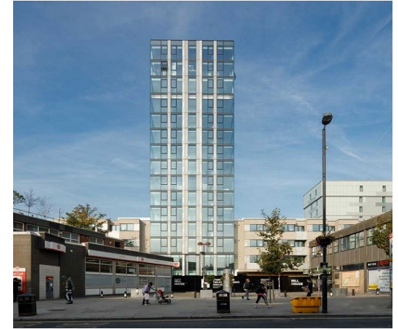
Fig. 4 Sympathetic tower refurbishment at Hill House (refurbishment), Archway, London, N19 5NA
