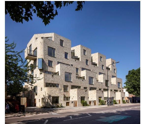
Fig. 5 Dynamic facade on 95 Peckham Road, London SE15 5FA
