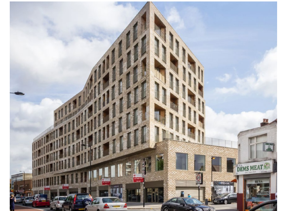
Fig. 5 Commercial ground floor below residential at Prowse Court, 74 Fore Street, Edmonton London N18 2FF
