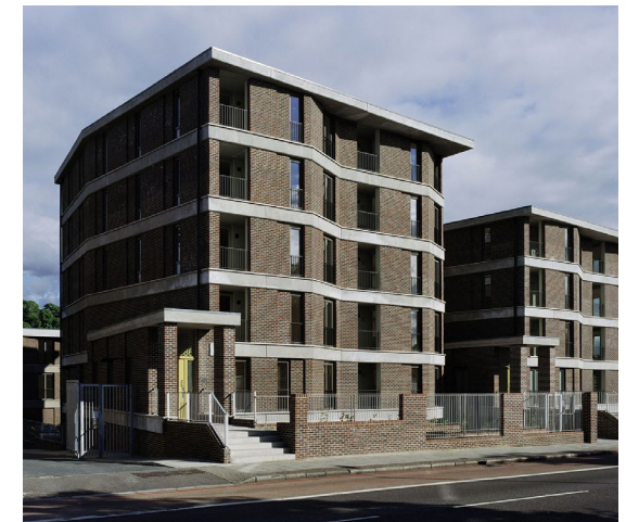
Fig. Set-back frontages at 5 384-386 Seven Sisters Road, Finsbury Park, London N4 2PQ
