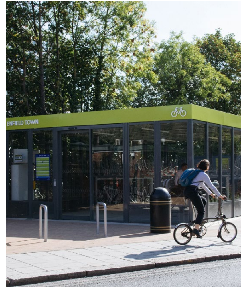
2. Cycle storage at Edmonton Green station, Enfield
