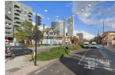
1. Bespoke lighting on Stratford High Street, Newham
