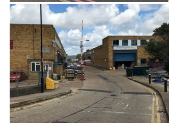
4. Poorly maintained retail frontages and industrial areas to the south (three above)
