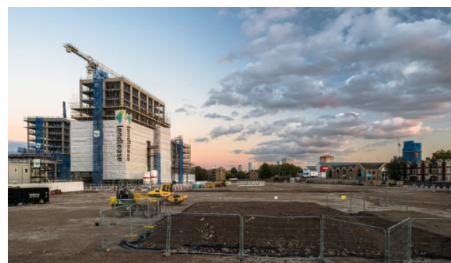
Photo 5: Timberyard Under Construction Source: LB Lewisham
