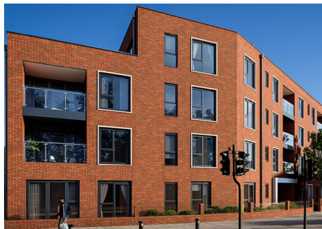
Photo 13: Former Sydenham Police Station Source: PA Housing
