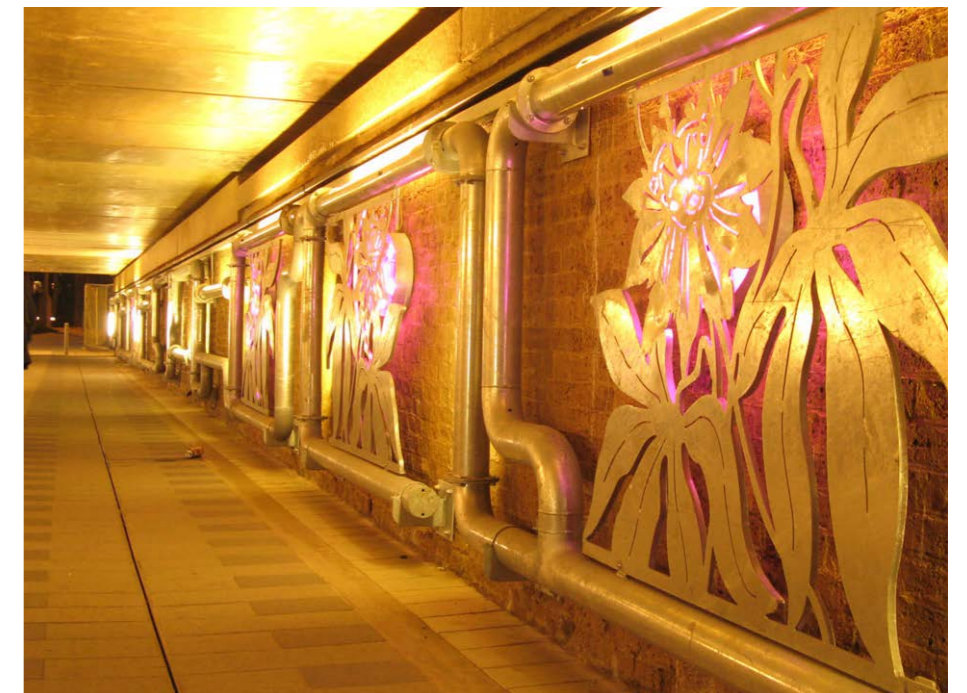
Fordham Park underpass, New Cross
