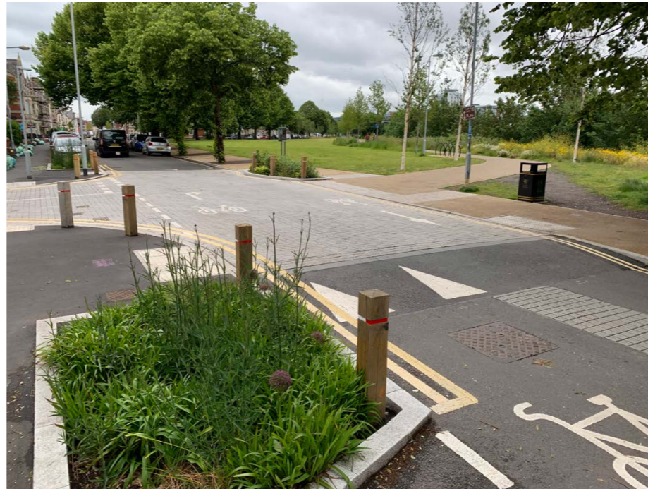
Taff Embankment, Cardiff
