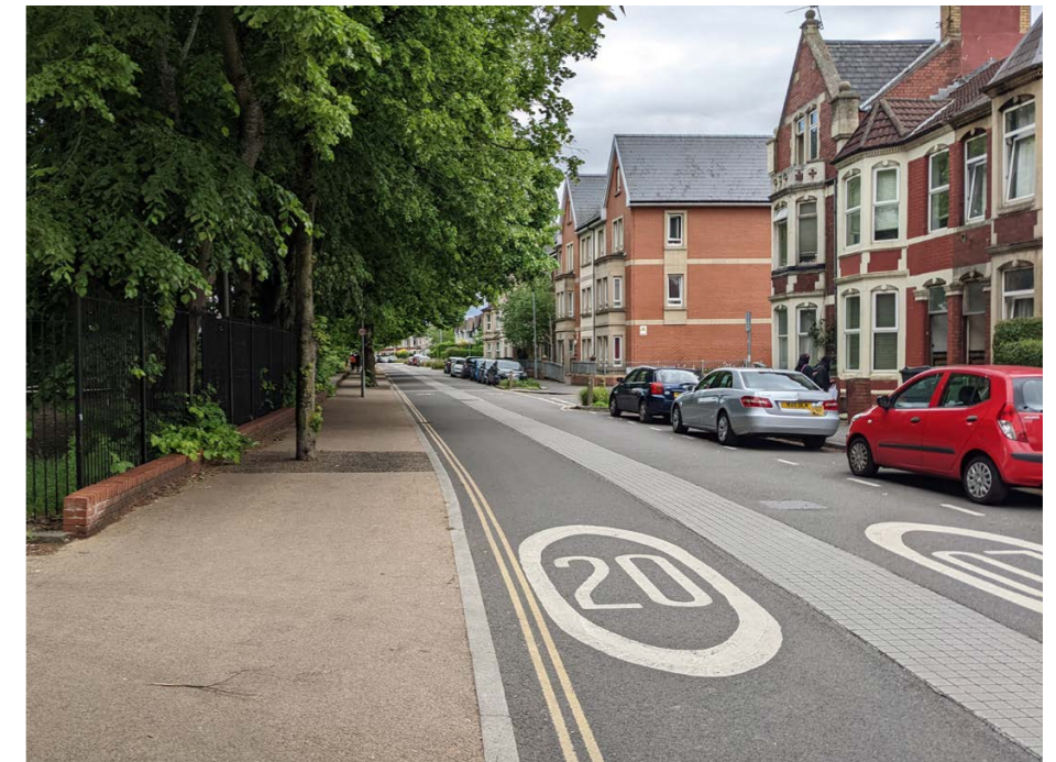
Taff Embankment, Cardiff
