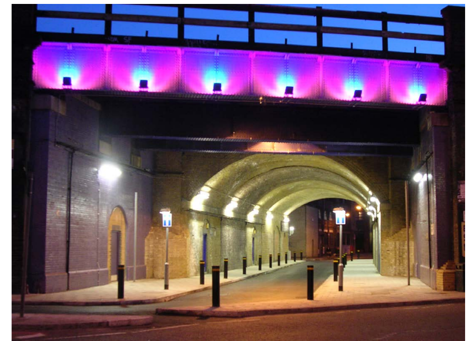
Light at the End of the Tunnel project, Tanner Street
