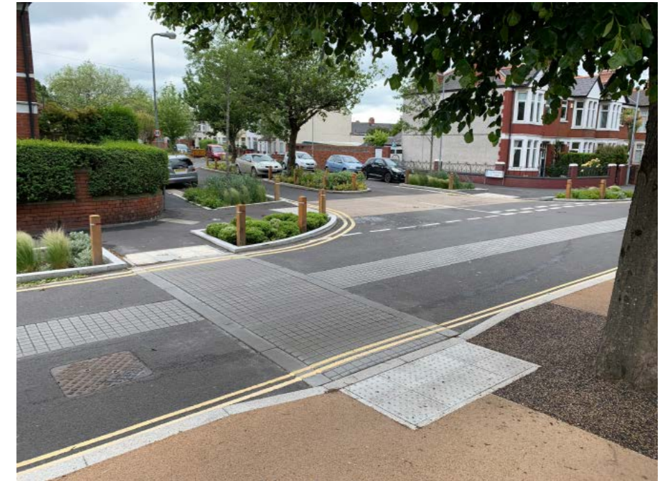
Taff Embankment, Cardiff
