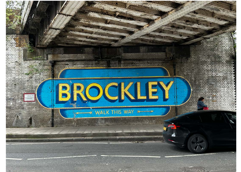
Underpass in Brockley
