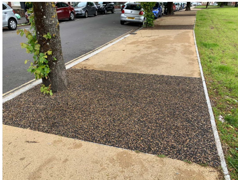
Footway tree pits
