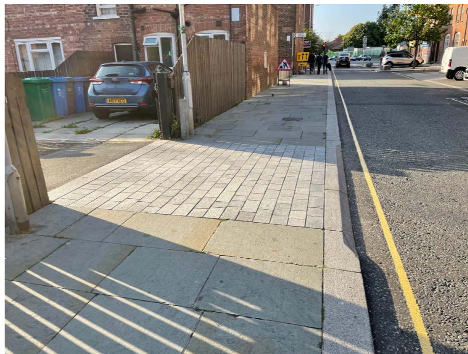
Chamfered edge kerb and smaller unit size surfacing
